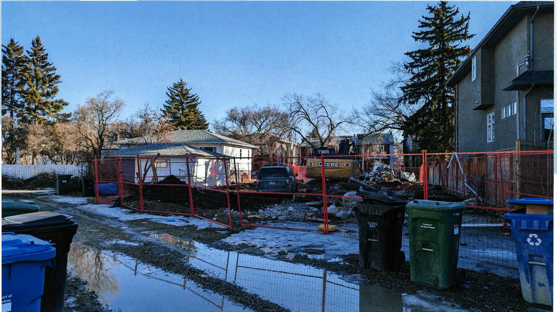
Site view from the lane
