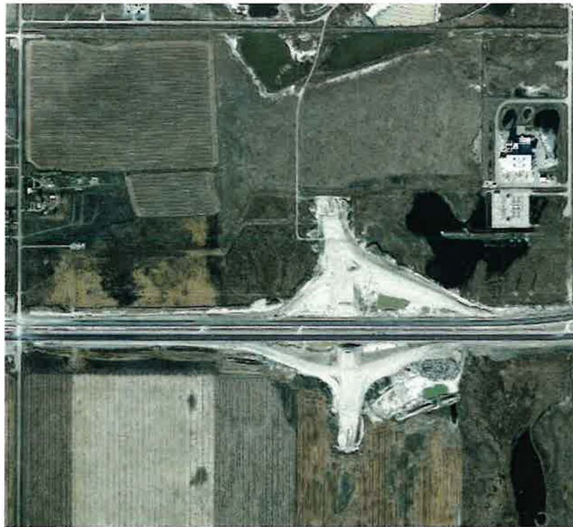
2007: Initial Stoney Trail Construction
