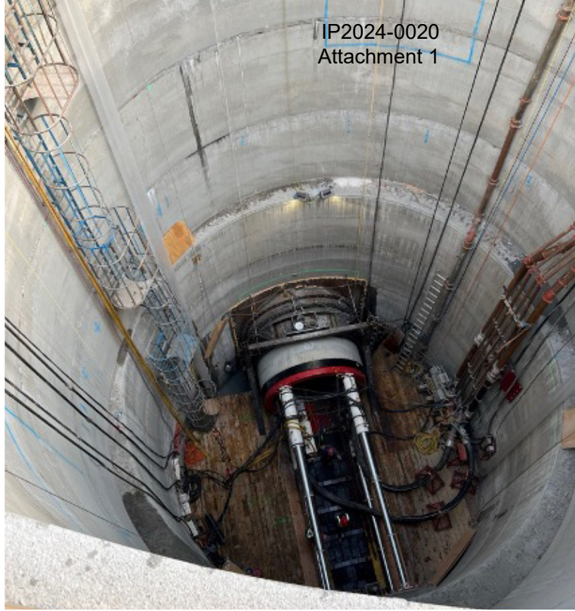
Upper Plateau Project: Launch shaft, used to lower micro-tunneler, pipe sections, hydraulic rams and to remove tunneling cuttings.
