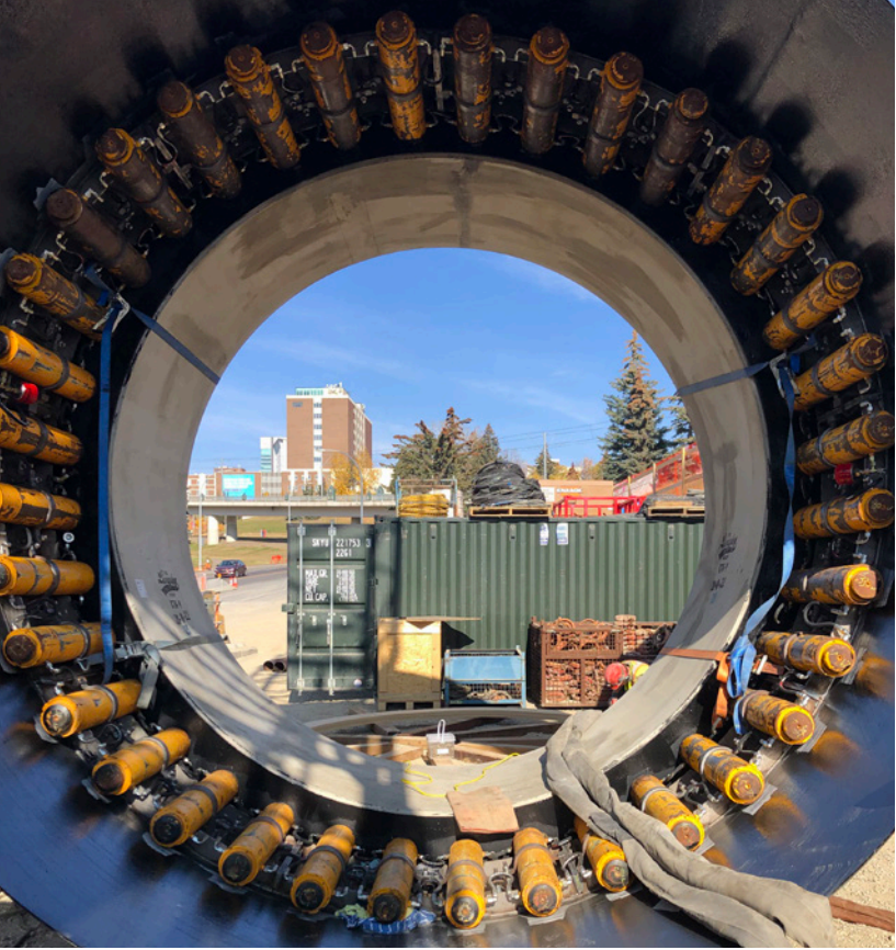
Upper Plateau Project: Launch shaft, used to lower micro-tunneler, pipe sections, hydraulic rams and to remove tunneling cuttings.
