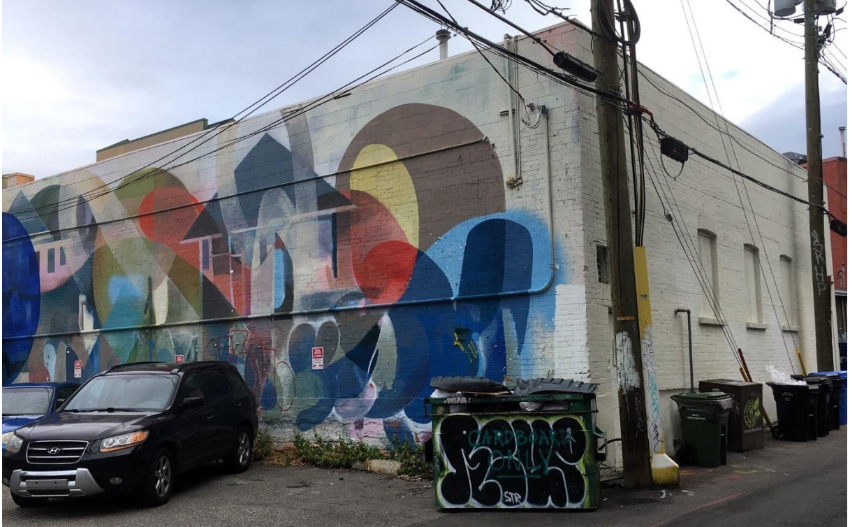
(Image 3.2: South and west façades showing rectangular form)
