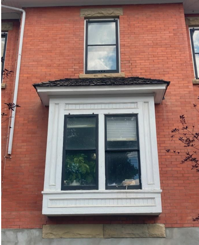
(Image 2.1 – Wood-panelled bay (oriel) window)
