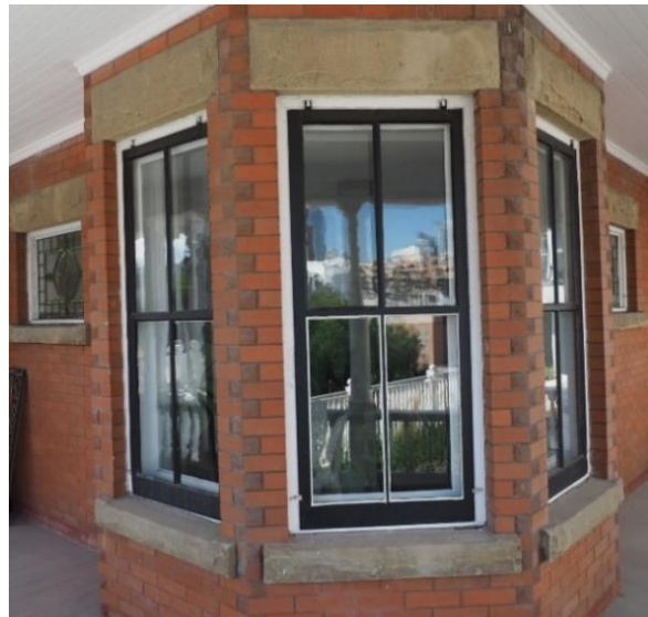
(Image 1.6 – Corner turret, showing examples of window with 4-pane wooden storm sash; rough-faced pitched brick detail at corners)
