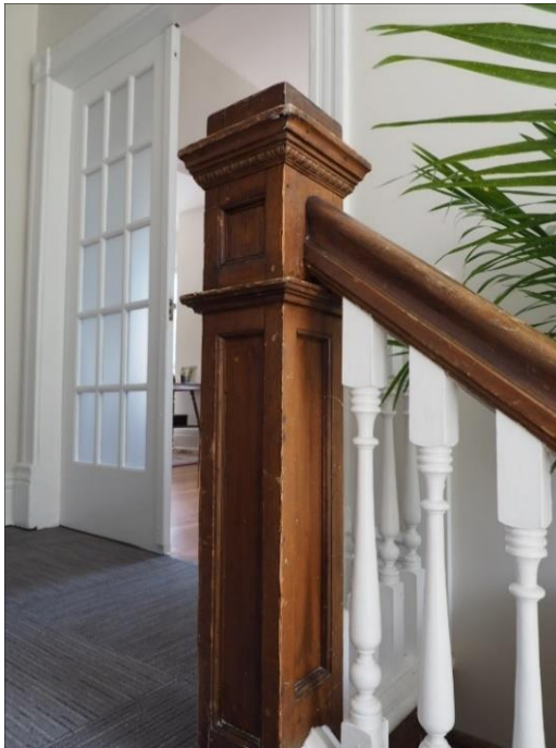
(Image 6.7 – Detail of second-storey newel post showing baluster and handrail profile)
