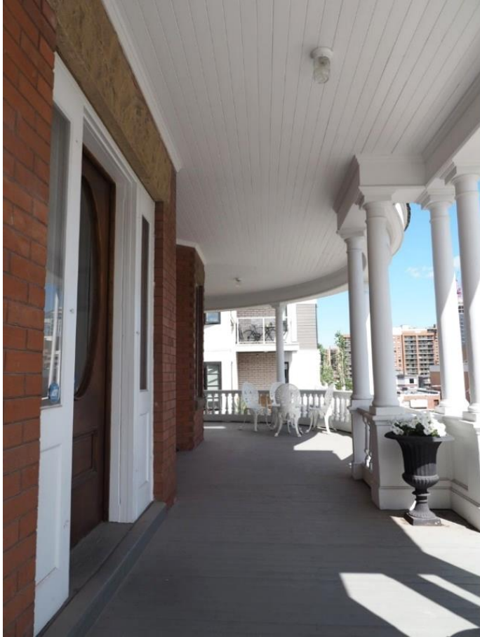
(Image 1.12 – Detail view of the veranda, looking north, showing tongue-and-groove ceiling)
