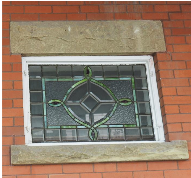
(Image 3.4 – Leaded glass window on north façade)
