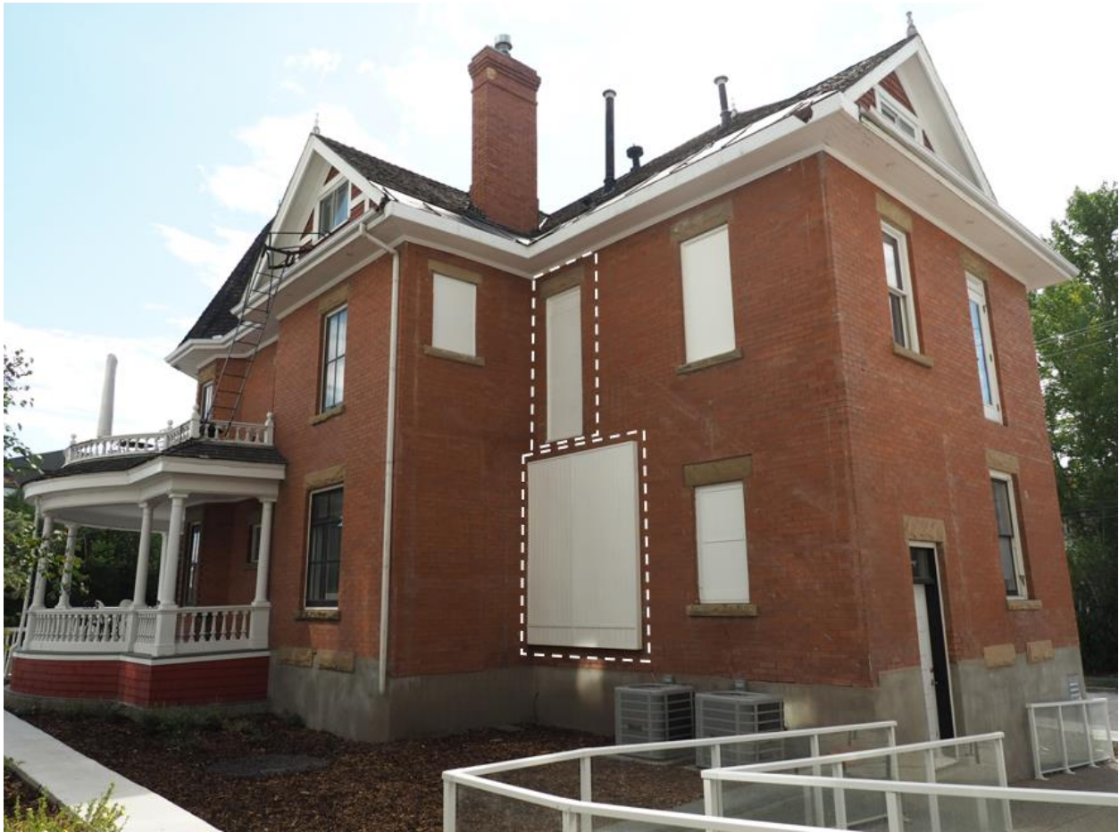
(Image 3.1 – Oblique view of the Nimmons Residence, looking southeast; dotted outlines indicate alterations to north façade from prior contemporary addition; all openings and historic windows, including those painted-over in white are regulated)
