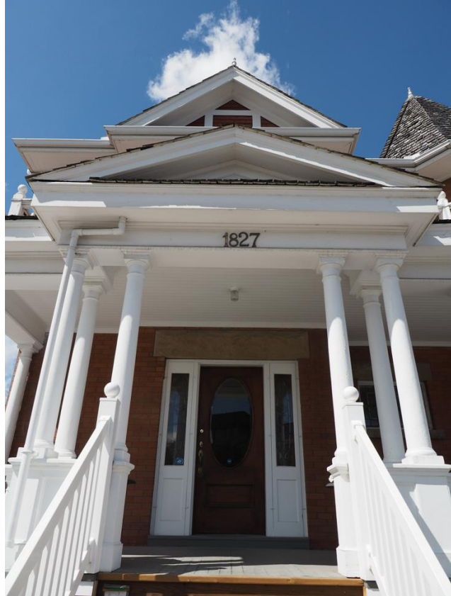
(Image 1.10 Detail of entrance pediment on veranda)
