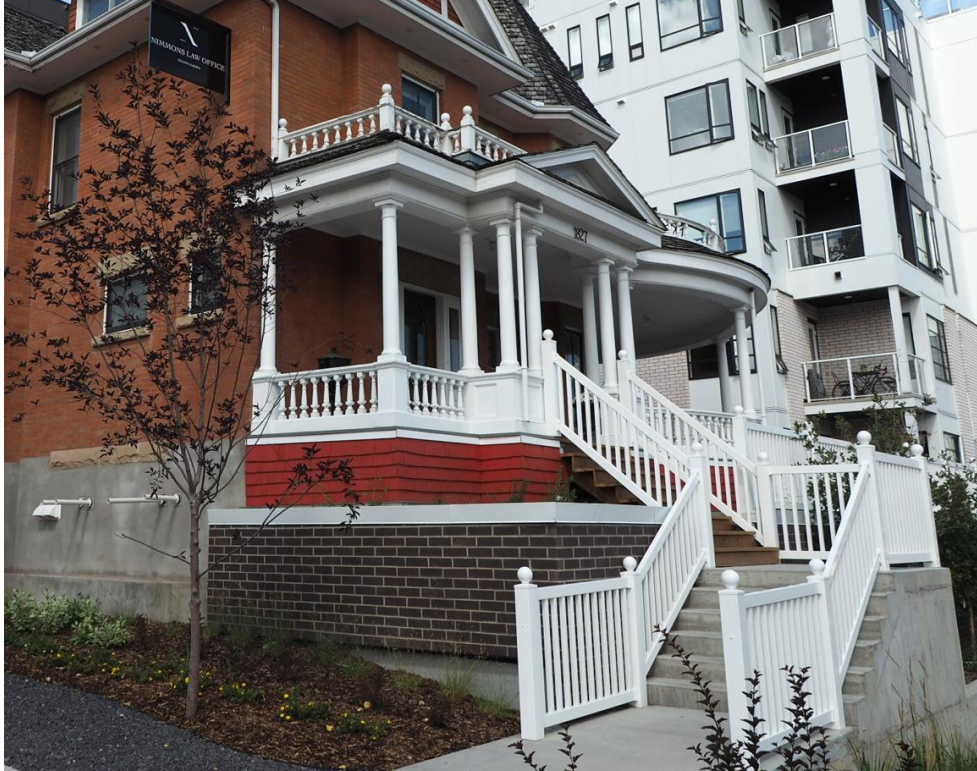
(Image 1.7 – Detail view of the veranda, looking northwest, showing balustrade and Tuscan-style columns; contemporary L-shaped stair accessing veranda is non-regulated)
