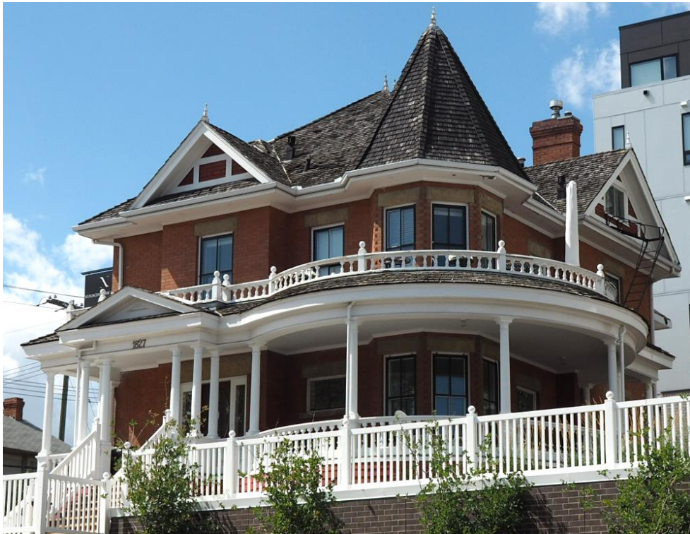
(Image 1.8 – Detail view of the veranda, looking southwest, showing balustrade and Tuscan-style columns)
