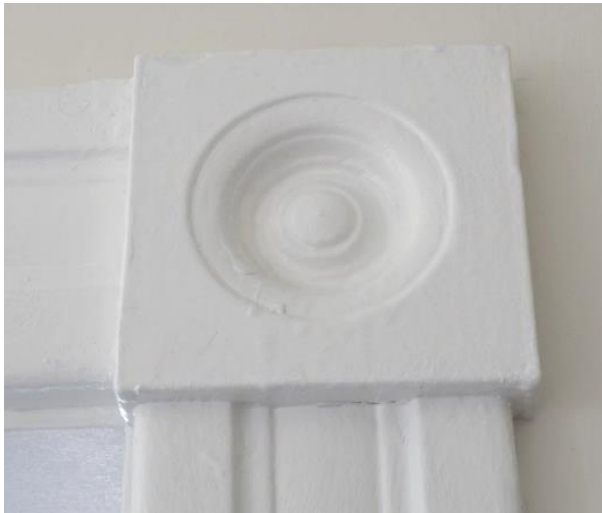
(Image 6.2 – Detail view showing example of doorway casing)
