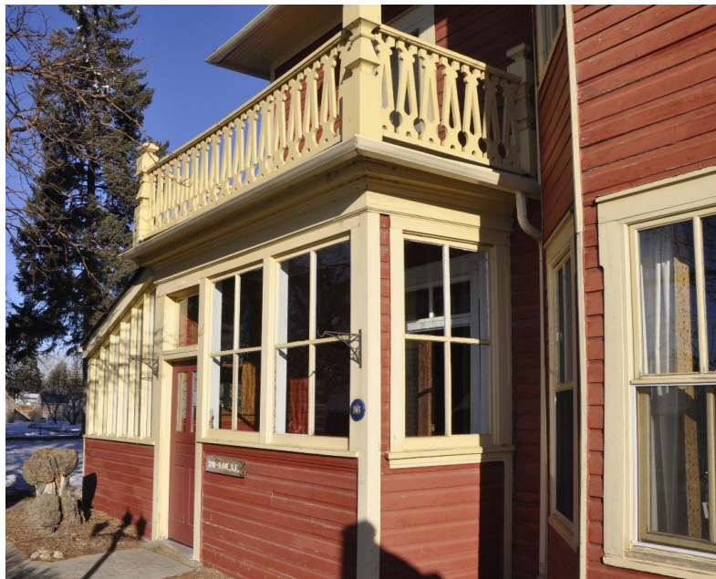
(Image 3.4: Oblique view of enclosed verandah, balcony and sunroom. Verandah exterior: East and south-facing 4-light double-assembly wooden window sashes evenly segmented by wooden mullions, heads and sills; transom window and door opening including wood casings)
