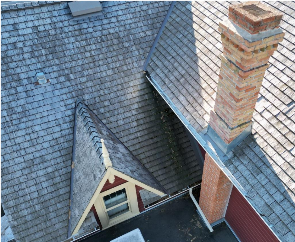
(Image 2.8: Original red brick chimney with heavily corbelled top. West-facing gable dormer with single-hung sash window can also be seen in this photo)
