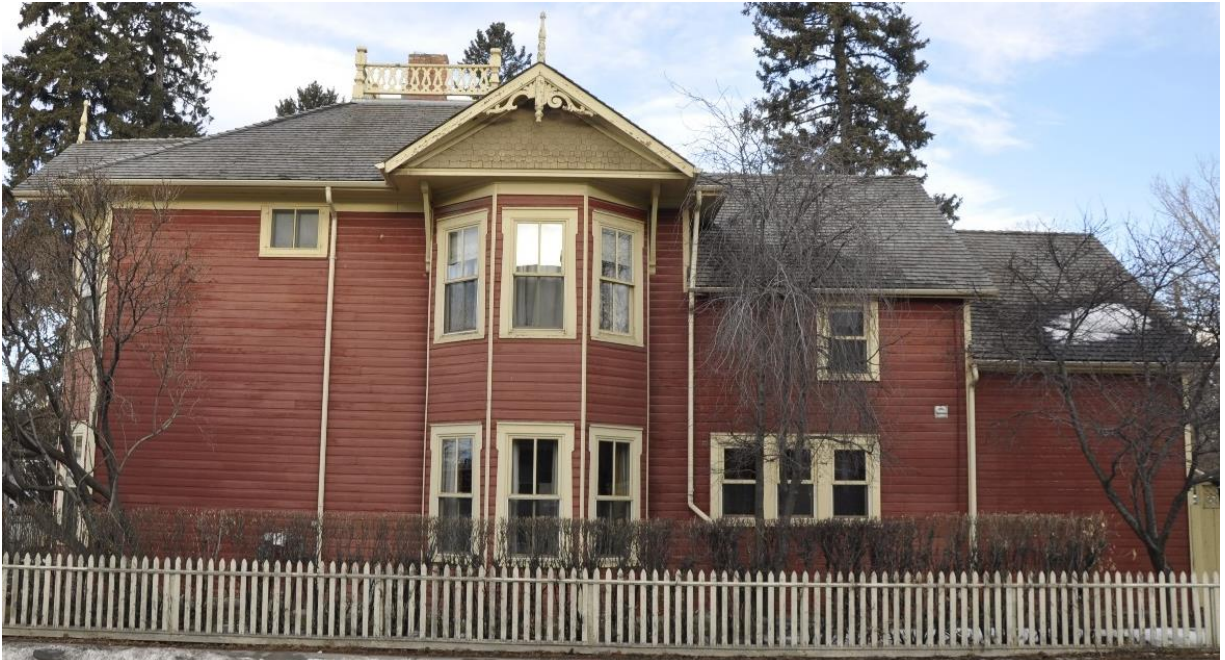
(Image 5.1: East façade showing projecting two-storey bay, widow's walk and Building Section 2)
