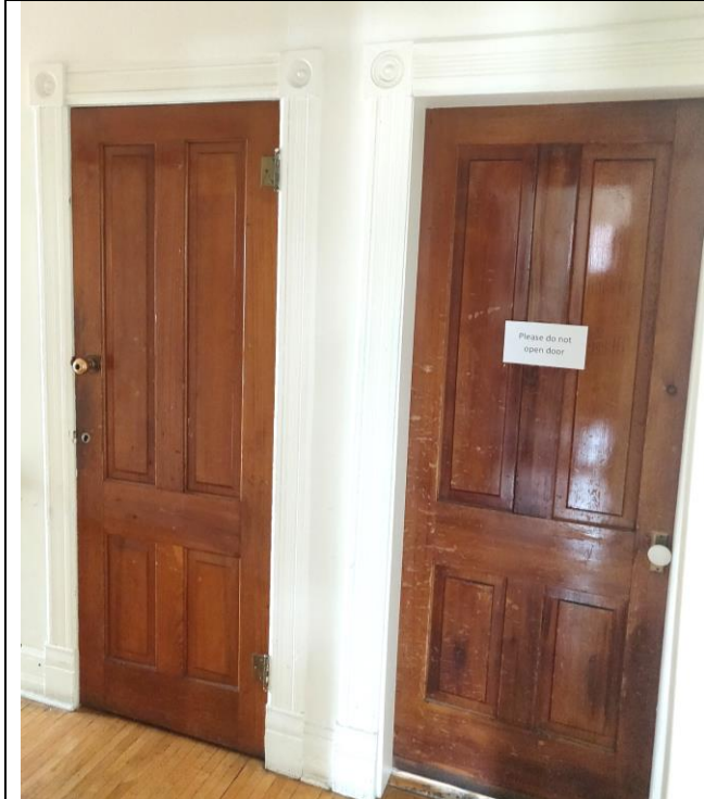
(Image 6.12: Example of wooden doors and profiled frames)
