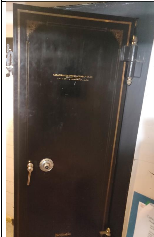
(Image 6.14: Vault door, located in basement)
