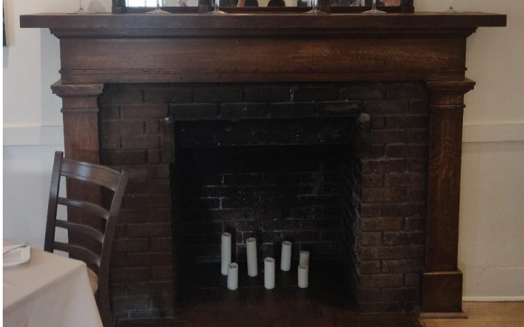
(Image 6.9: Brick fireplace with tiled hearth, profiled wooden mantle and surround)
