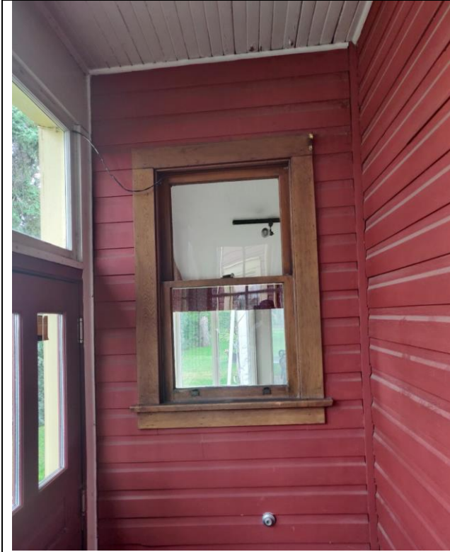
(Image 3.5: West-facing 1-over-1 wooden hung sash, wooden casing and sill inside enclosed verandah)
