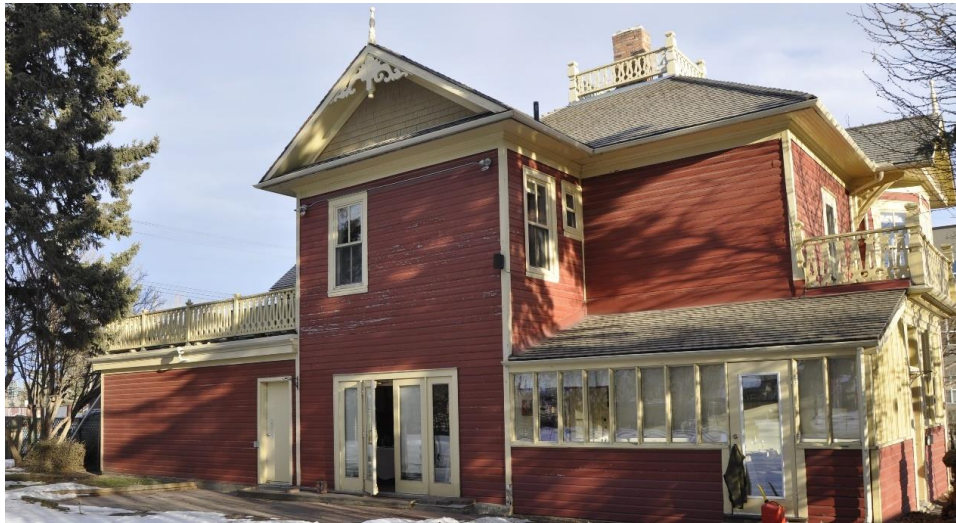
(Image 4.1: Building Section 1 – West façade showing sunroom addition with narrow eaves and projecting two-storey addition with pedimented gable clad in wooden square shingles, projecting verge with profiled wooden frieze, tongue-and-groove wooden soffits, plain wooden bargeboard, decorative scrollwork and finial)
