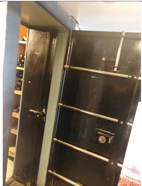
(Image 6.15: Vault door, located in basement)
