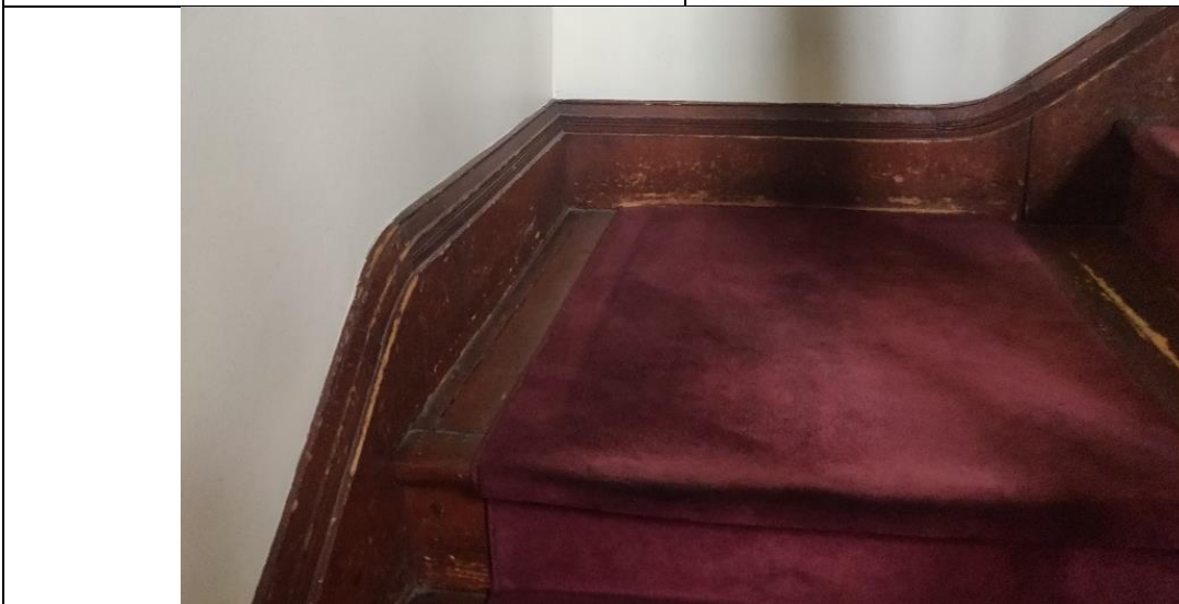
(Image 6.3: Example of staircase's profiled wooden baseboard and hardwood flooring)
