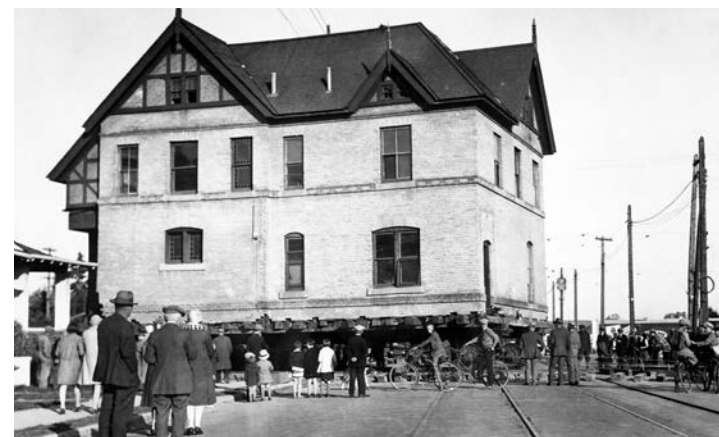
John R. Costigan's house, later occupied by Col. Sam Steele, being moved across 17 Avenue SW from Beltline to its present site in Mission, 1928. W.J. Oliver, photographer. Glenbow Library and Archives Collection, Libraries and Cultural Resources Digital Collections, University of Calgary, CU193180
