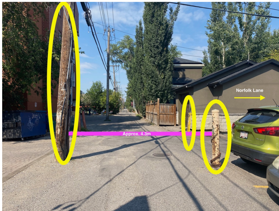
Figure 4: Rear laneway looking west from 10th ST - barriers and challenges for vehicles to turn east from Norfolk Lane
