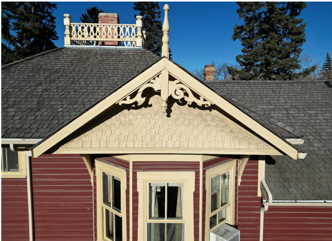
(Image 2.3: Example of one of two projecting two-storey bays with angled gable pediment, clad in wooden octagonal and square shingles, projecting verge with profiled wooden frieze, tongue-and-groove wooden soffits, plain wooden bargeboard, decorative scrollwork and finial, and supported by wooden brackets with decorative panel inlay)
