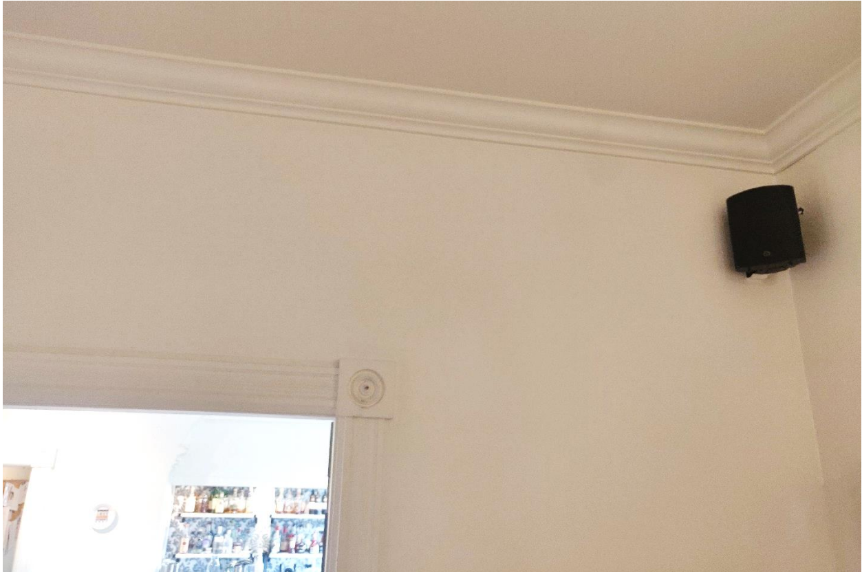
(Image 6.4: Example of crown moulding on ceiling. Partial door frame casing visible)
