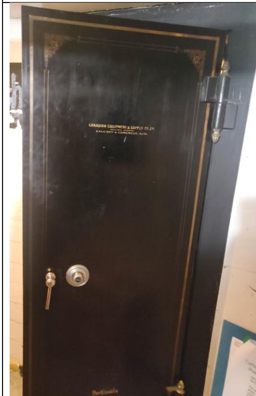
(Image 6.14: Vault door, located in basement)
