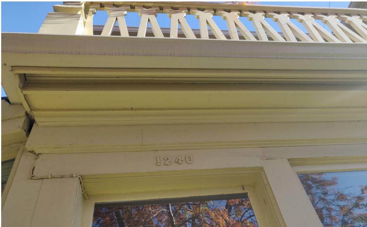
(Image 2.5: South-facing enclosed verandah: eaves, built-up wooden soffit, profiled wooden frieze and plain wooden fascia)
