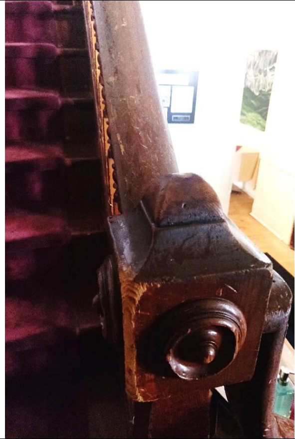
(Image 6.7: Carved fir newel posts and balusters on stairway)
