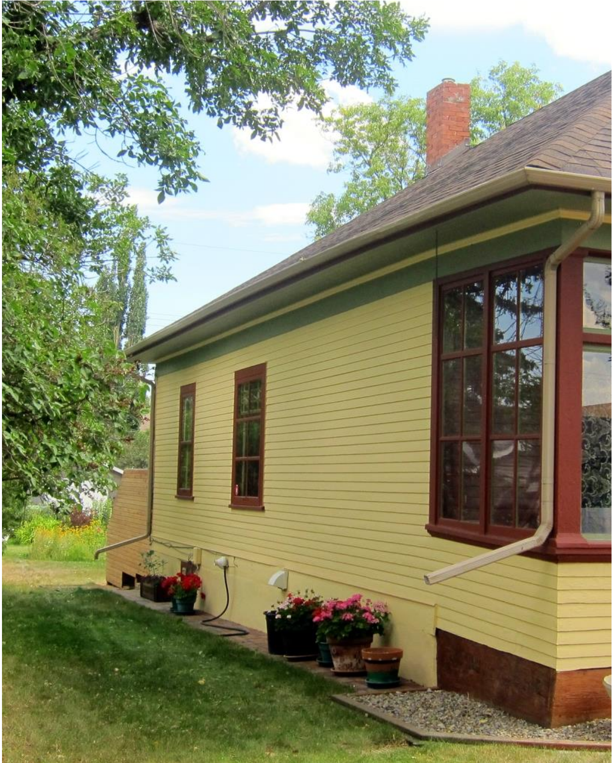
(Image 1.2: North façade showing six-light double-assembly wooden window sashes evenly segmented by wooden mullions, posts, heads and sills (enclosed verandah); 1-over-1 wooden window sash, wooden mullions, heads and sills; beveled-wood siding; moulded frieze, plain wooden fascia, overhanging eaves. Note: storm windows are not regulated)
