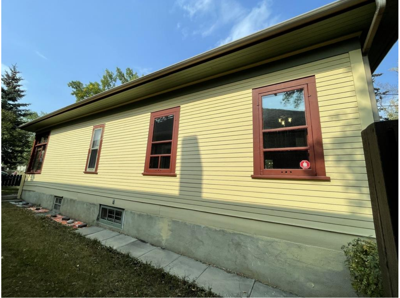
(Image 1.6: South façade showing single assembly 1-over-1 wooden window sash including 2, 3 and 4-light wood storm window sashes, wooden mullions, heads, and sill; beveled-wood siding. Note: storm windows are not regulated)
