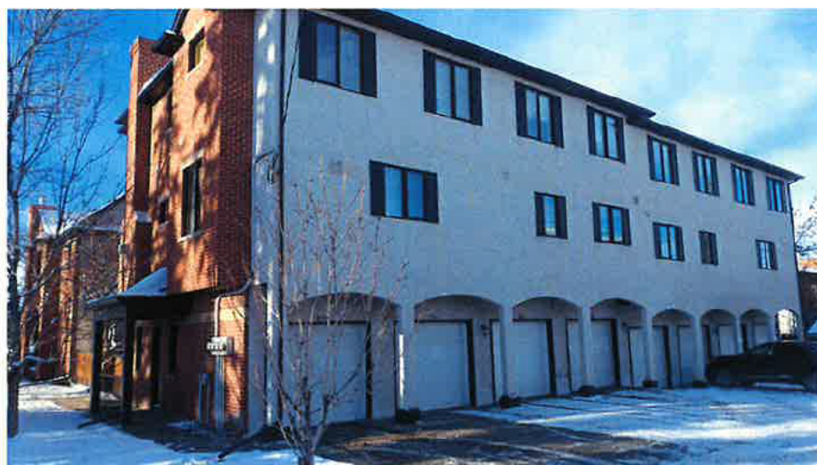
Killarney 29St 18Ave SW 2 lot parking arrangement north west view
