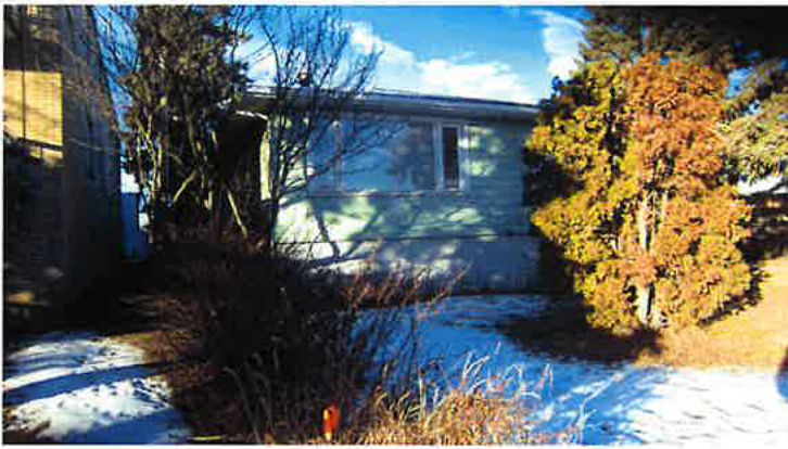
#1 10:05 am, Dec. 30. 2023 1735 26 St SW south/east side roof in shade
