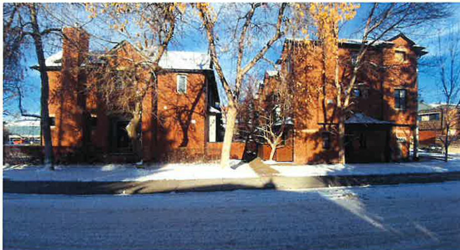
Killarney 29St 18Ave SW court yard space north view
