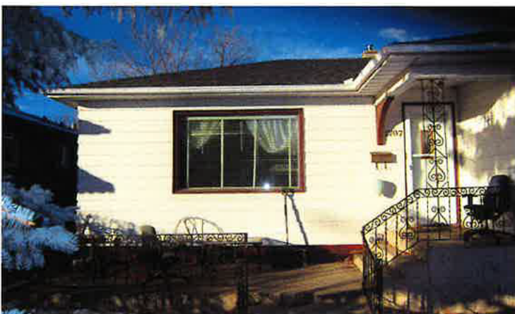
#4 10:00 am, 30. Dec. 2023 1707 26 ST SW east side roof in sun
