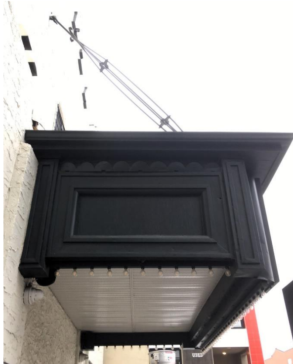
(Image 3.4: Detailed side image of suspended marquee)
