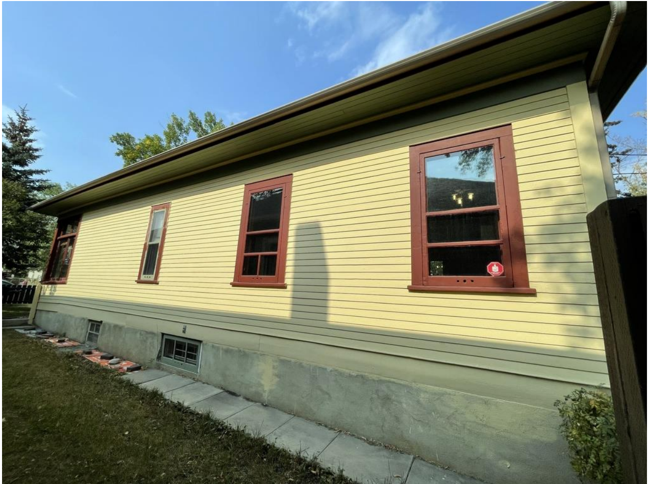
(Image 1.6: South façade showing single assembly 1-over-1 wooden window sash including 2, 3 and 4-light wood storm window sashes, wooden mullions, heads, and sill; beveled-wood siding. Note: storm windows are not regulated)
