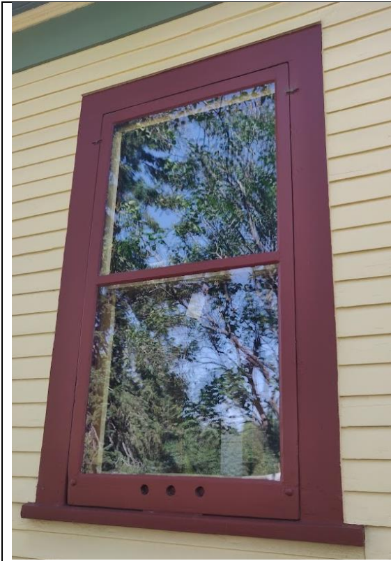
(Image 1.7: Example of typical 1-over-1 wooden window sash. Note: storm window is not regulated)
