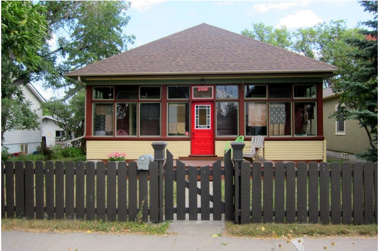
(Image 1.1: West façade with full-width enclosed verandah; single-assembly and triple-assembly wooden window and transom sashes evenly segmented by wooden mullions, posts, heads and sills, central entry door; steeply-pitched hipped roof)
