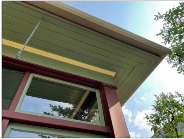
(Image 1.3: Overhanging eaves, wooden tongue-and-groove soffits, moulded wooden frieze, plain wooden fascia)
