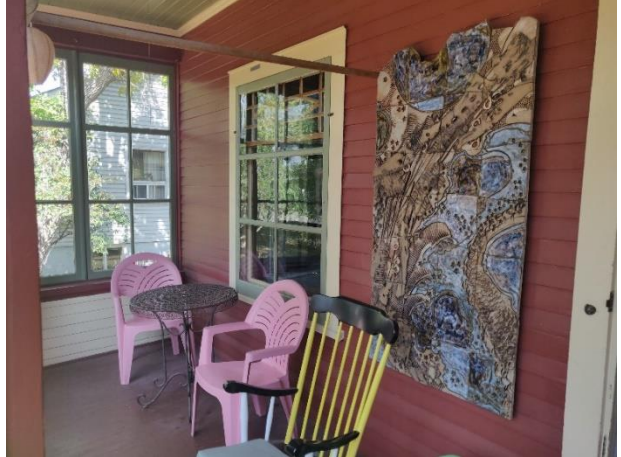
(Image 1.4: Interior of enclosed verandah showing exterior north-facing six-light double-assembly windows: wooden tongue-and-groove ceiling, beveled wood siding on interior walls, crown moulding, wooden plank flooring; 1-over-1 wooden hung-sash windows including 6-light wood storm window sashes, wooden mullions, heads, and sills)
