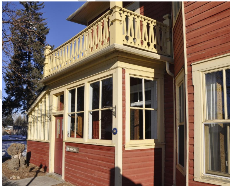
(Image 3.4: Oblique view of enclosed verandah, balcony and sunroom. Verandah exterior: East and south-facing 4-light double-assembly wooden window sashes evenly segmented by wooden mullions, heads and sills; transom window and door opening including wood casings)
