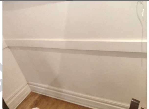
(Image 6.2: Example of chair rail and profiled wooden baseboards)
