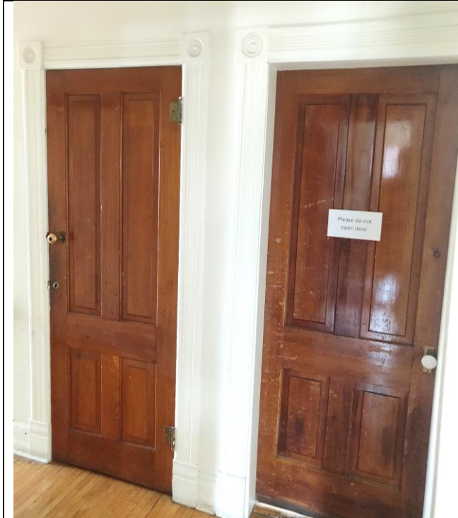
(Image 6.12: Example of wooden doors and profiled frames)
