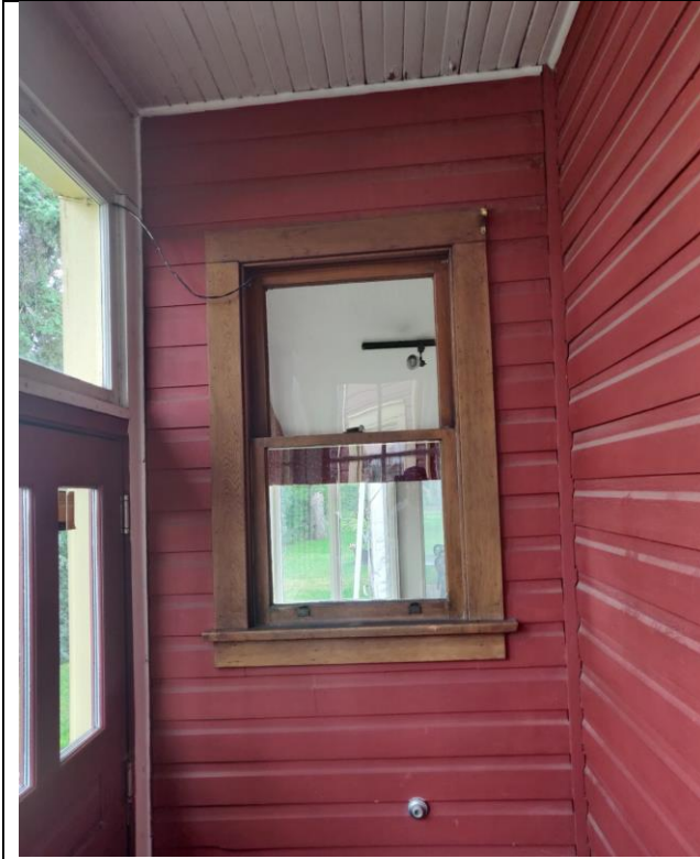
(Image 3.5: West-facing 1-over-1 wooden hung sash, wooden casing and sill inside enclosed verandah)
