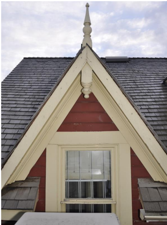
(Image 2.7: West-facing gabled dormer clad in wooden siding, projecting verges with profiled wooden frieze, tongue-and-groove wooden soffits, plain wooden bargeboard, finial)
