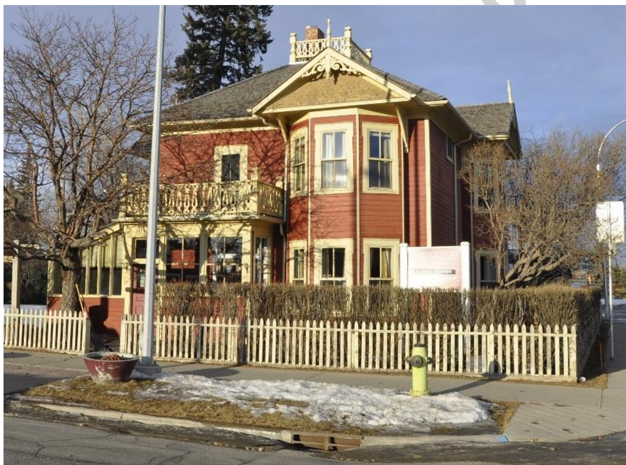
(Image 3.1: South façade showing pedimented gable over projecting two-storey bay, enclosed verandah, balcony and widow's walk)
