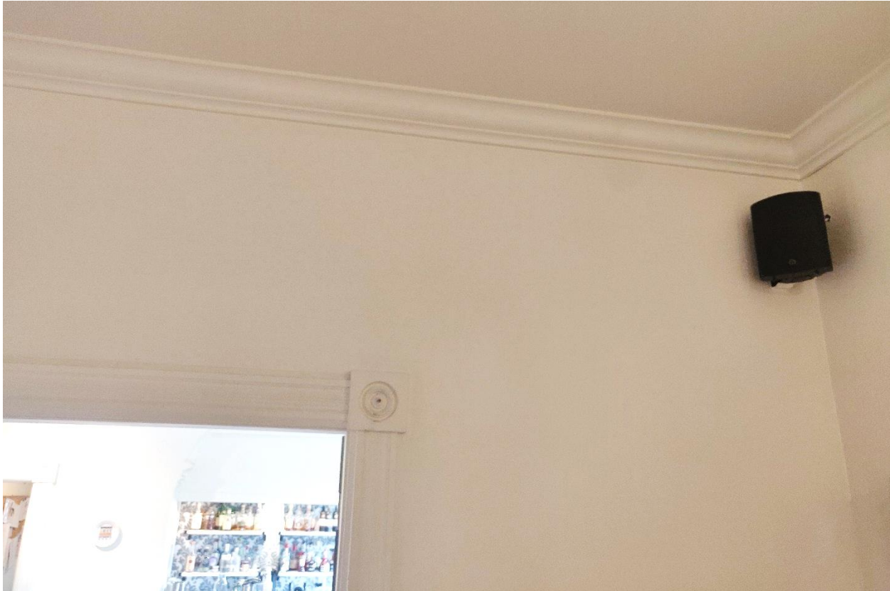
(Image 6.4: Example of crown moulding on ceiling. Partial door frame casing visible)
