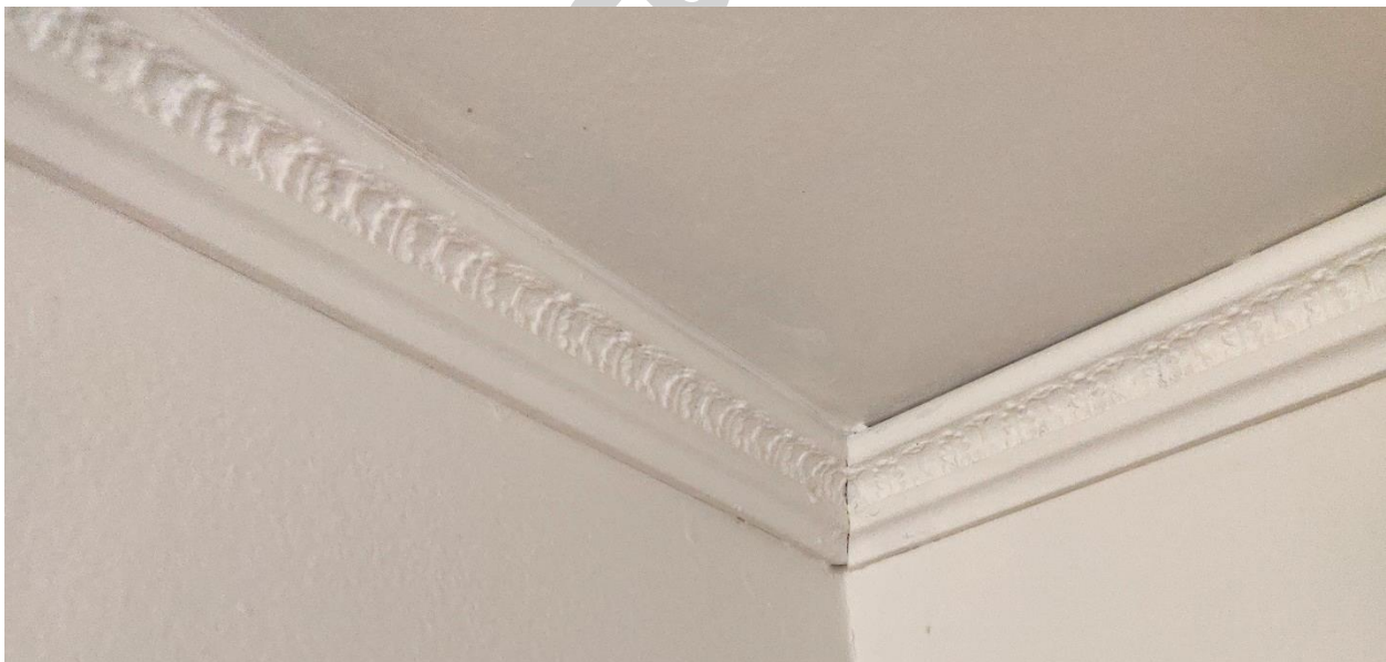
(Image 6.5: Another example of crown moulding with different articulation)
