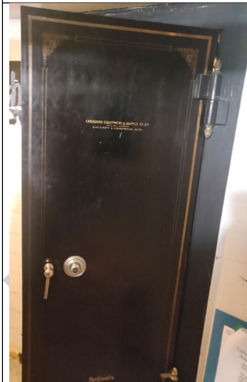
(Image 6.14: Vault door, located in basement)
