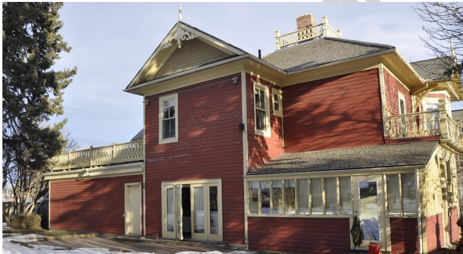
(Image 4.1: Building Section 1 – West façade showing sunroom addition with narrow eaves and projecting two-storey addition with pedimented gable clad in wooden square shingles, projecting verge with profiled wooden frieze, tongue-and-groove wooden soffits, plain wooden bargeboard, decorative scrollwork and finial)
