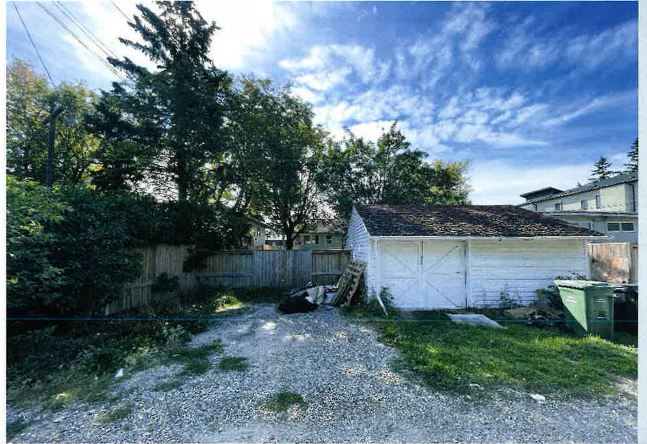
1212 - 20 Avenue NW from the lane
