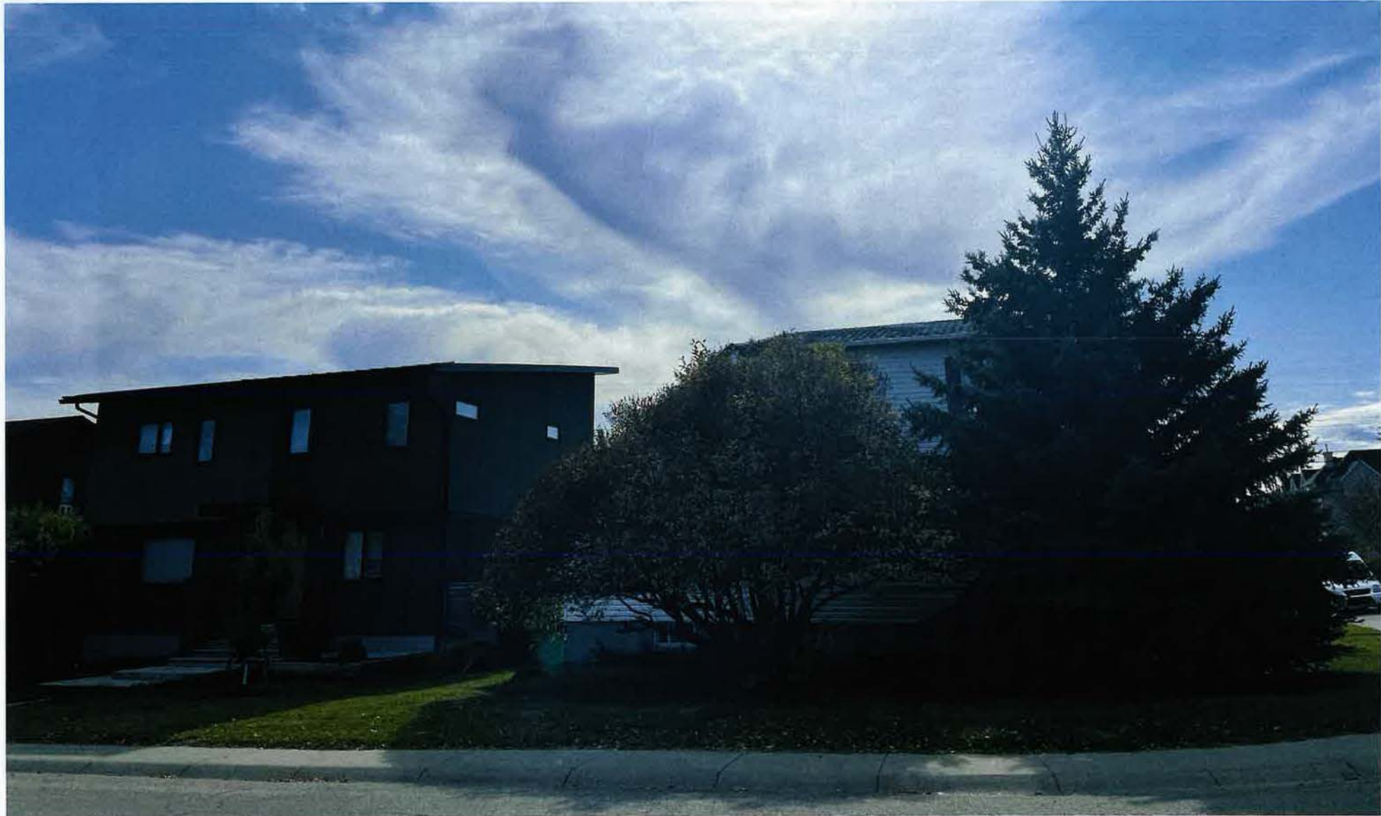
Looking south from 21 Avenue NE
