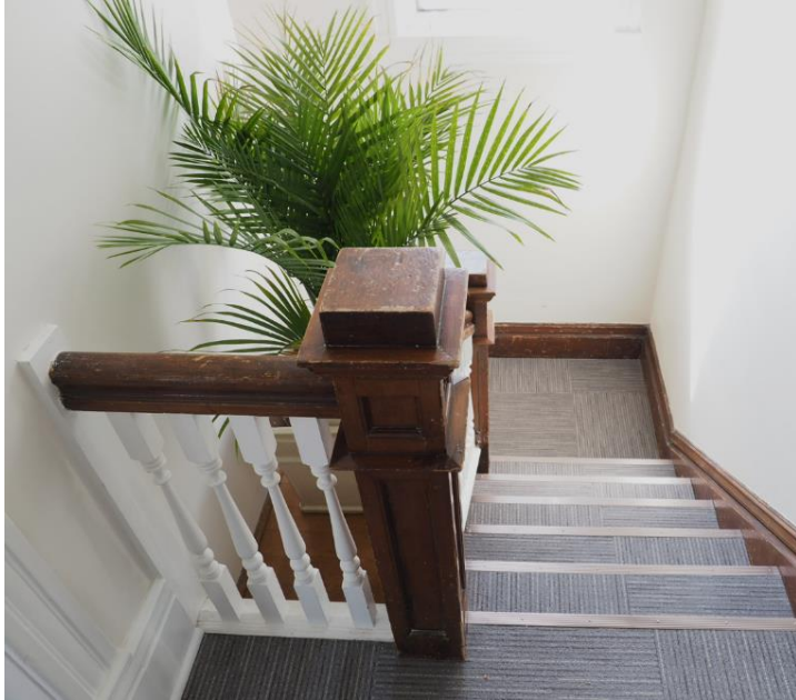
(Image 6.5 – Main staircase, looking from top of stairs, showing second-storey newel post)
