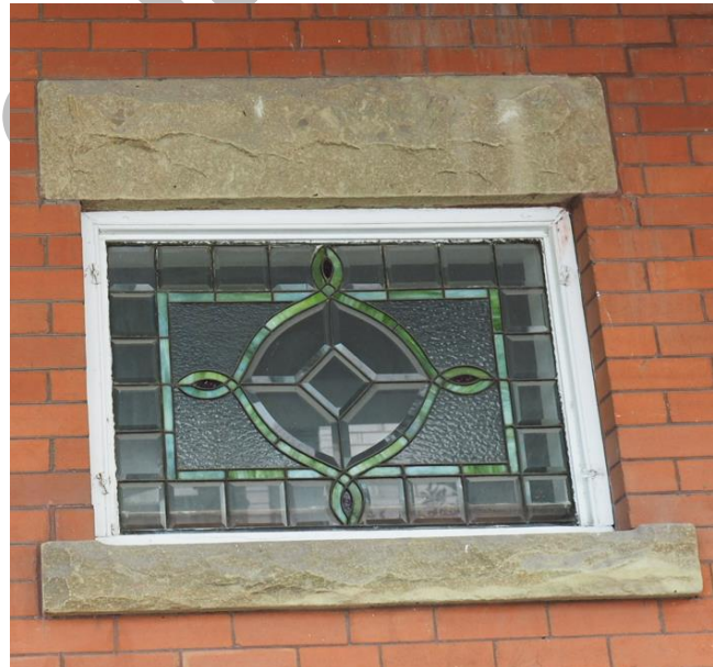
(Image 3.4 – Leaded glass window on north façade)
