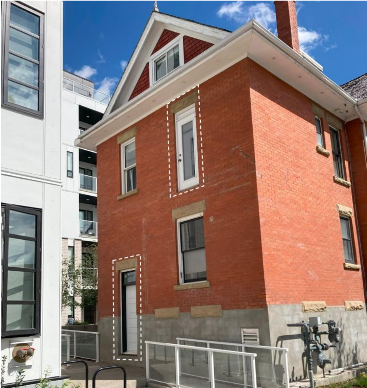
(Image 4.1 – Oblique view of the Nimmons Residence, looking northeast; dotted outlines indicate alterations to west façade from prior contemporary addition)
