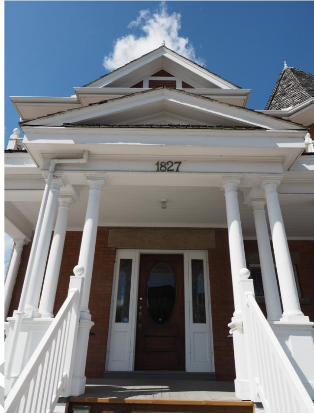
(Image 1.10 Detail of entrance pediment on veranda)
