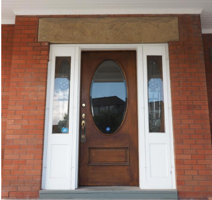
(Image 1.3 – Main entrance, showing doorway assembly)
