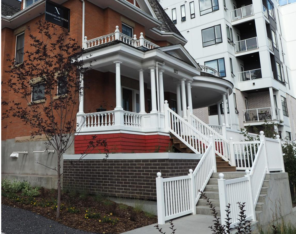
(Image 1.7 – Detail view of the veranda, looking northwest, showing balustrade and Tuscan-style columns; contemporary L-shaped stair accessing veranda is non-regulated)
