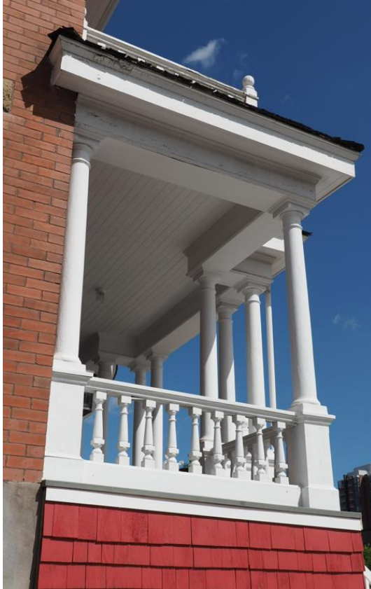
(Image 1.9 – South facade of the veranda, showing column detail and tongue-and-groove ceiling)
