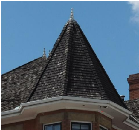
(Image 5.0 – Detail view of turret roof)
