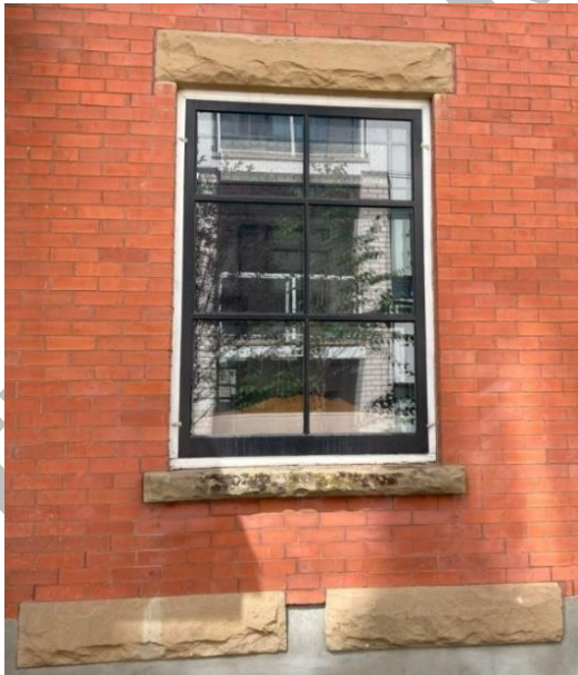
(Image 3.3 – Large north façade window with decoratively patterned upper sash)
