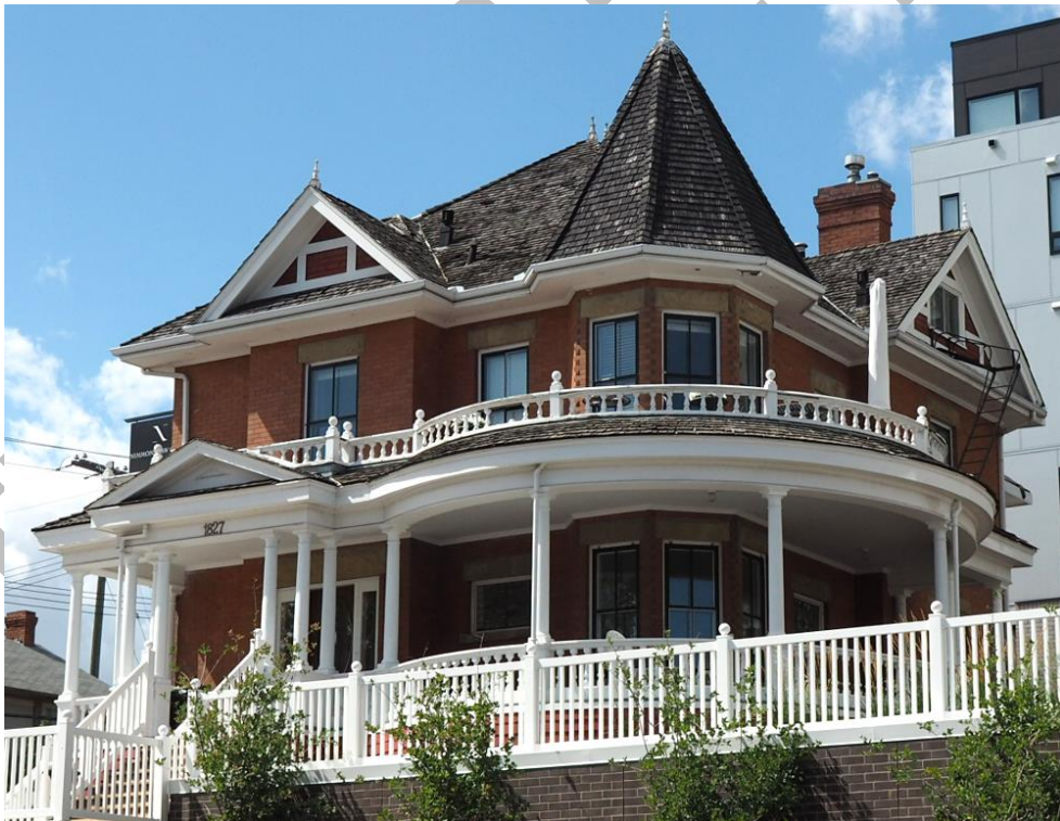
(Image 1.8 – Detail view of the veranda, looking southwest, showing balustrade and Tuscan-style columns)
