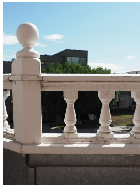
(Image 1.14 – Detail view of balustrade at balcony level, looking east)
