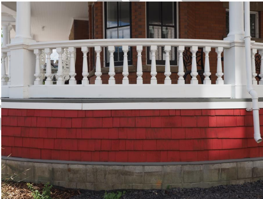
(Image 1.11 – Detail view of veranda skirt at northeast corner of the Nimmons Residence, showing baluster and column profile)
