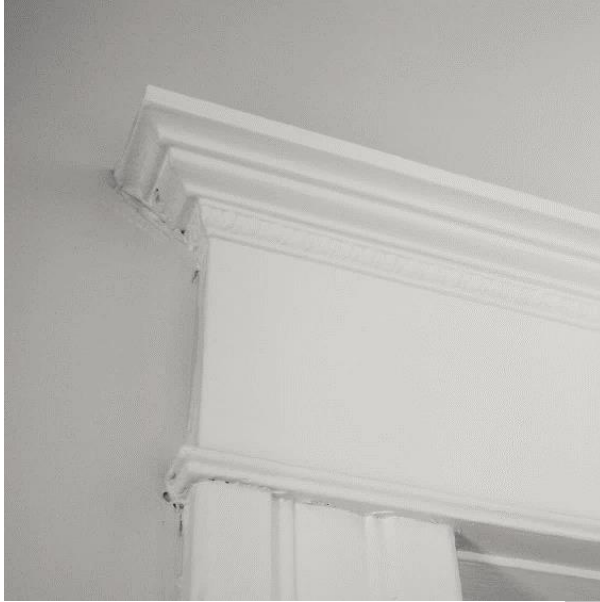
(Image 6.0 – Detail view showing more-ornate window casing entablature)
