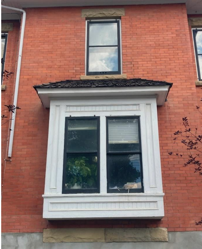
(Image 2.1 – Wood-panelled bay (oriel) window)
