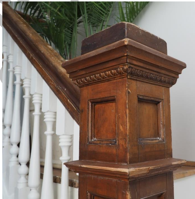
(Image 6.8 – Detail showing newel post at landing between first and second storeys)
