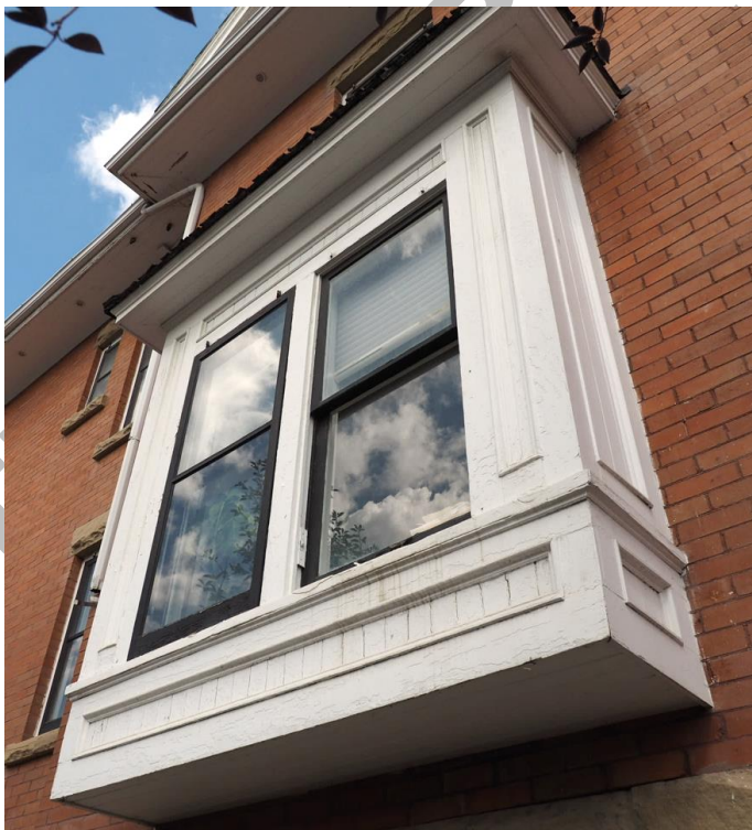
(Image 2.2 – Oblique view of Wood-panelled bay (oriel) window)
