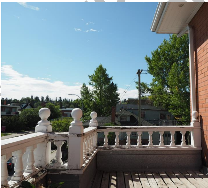
(Image 1.13 – Balustrade at balcony level, looking south)
