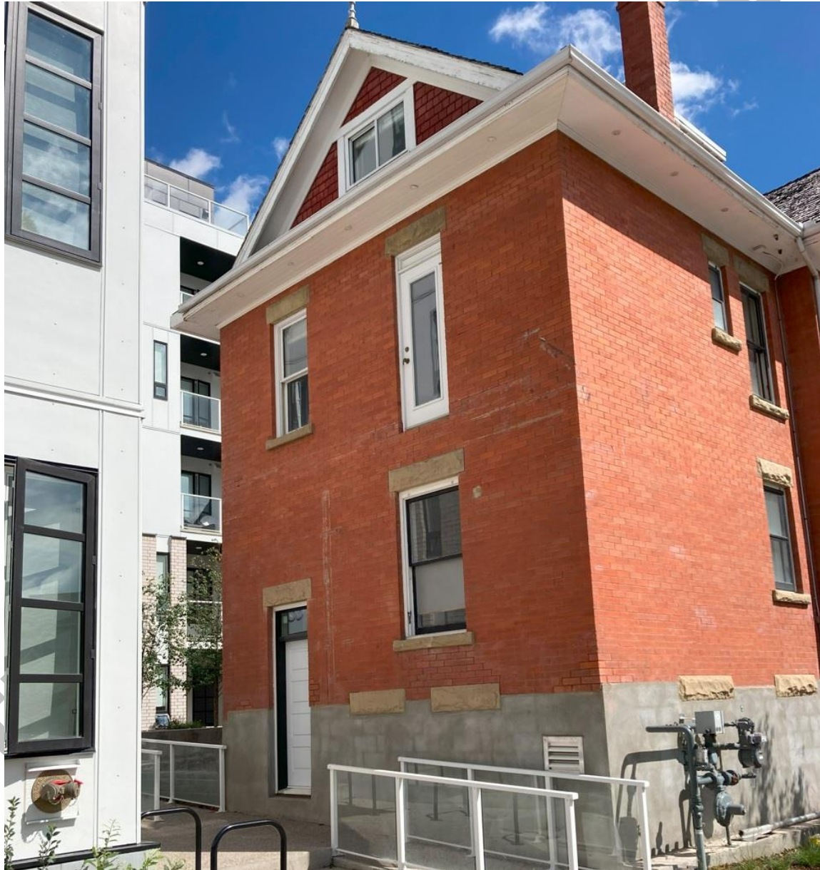
(Image 4.0 – Oblique view of the Nimmons Residence, looking northeast)
