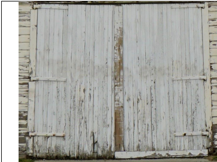
Image 2.2: Central wood double-doors and hardware
