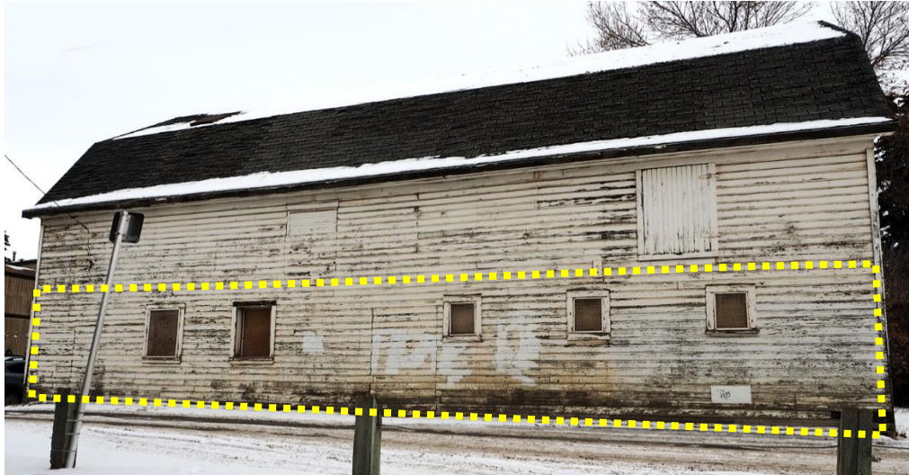
(Image 3.2: South façade; fenestration and existing windows on the first story as outlined in dotted lines are not regulated)
