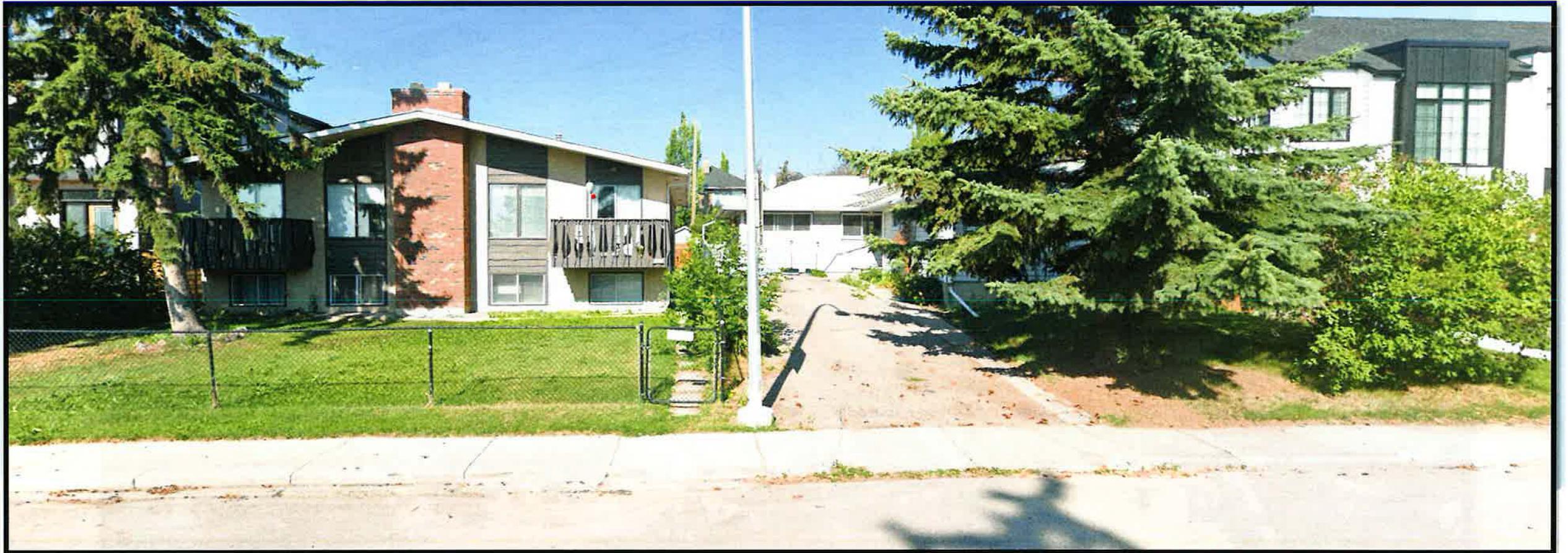
View from site looking WEST on 16 Street SW
