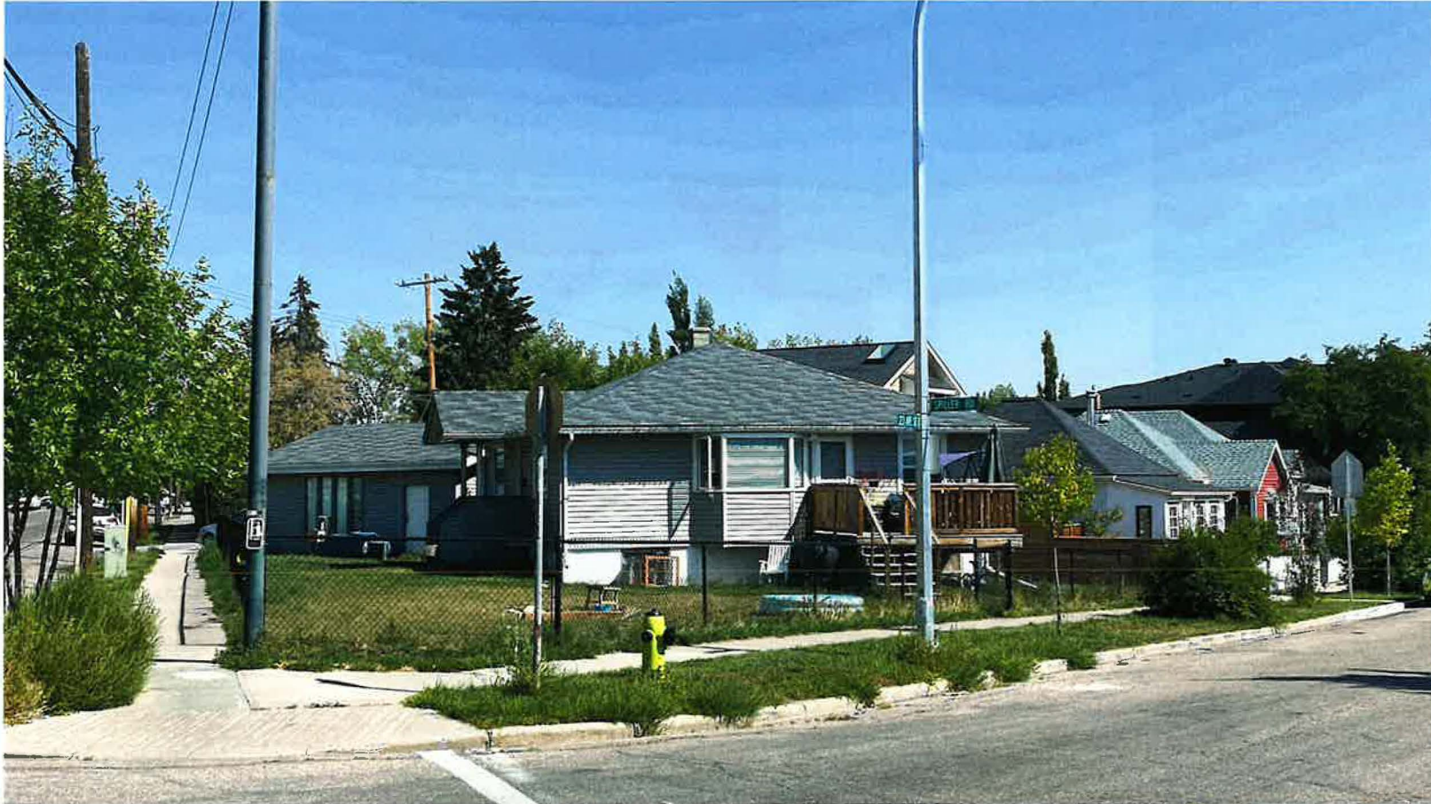
Front View from the corner of Spiller Road and 23 Avenue SE
