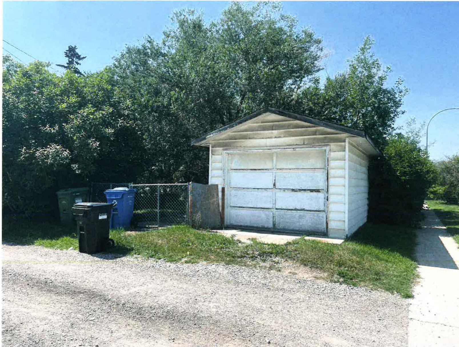
View from Rear Lane
