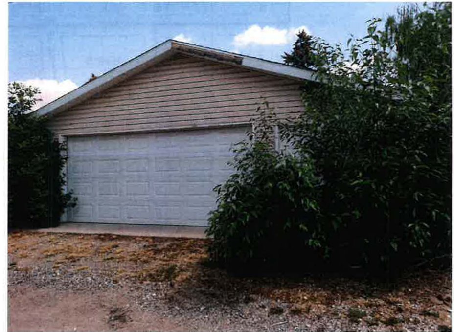
Garage – from Lane
