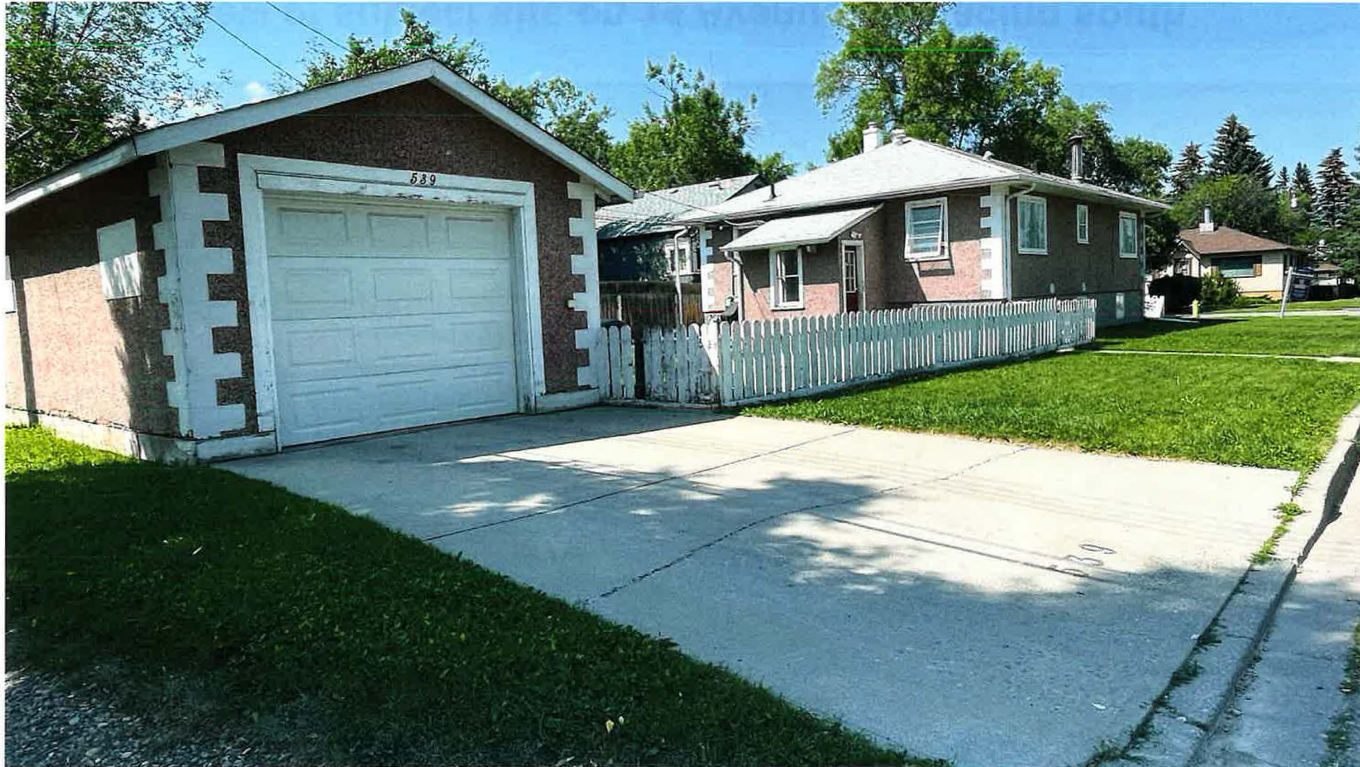
View of subject site on 5 Street NE, facing north
