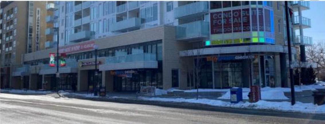
Figure 4: The existing Mary Brown's restaurant demonstrates how the Theodore's built form creates visually distinct store fronts with each commercial bay, despite being occupied by a single use.
