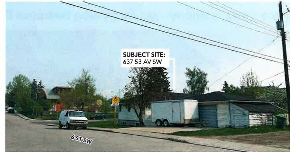
Looking northeast from 6 ST NW
