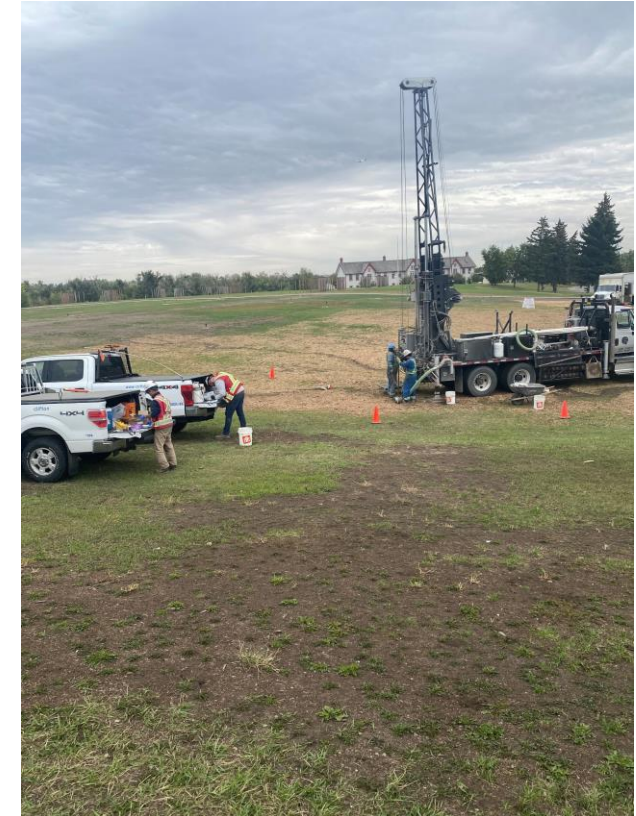
September 2023 Drilling for Geotechnical and Environmental Assessments
