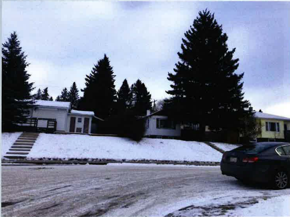
Front yard of subject site facing southwest
