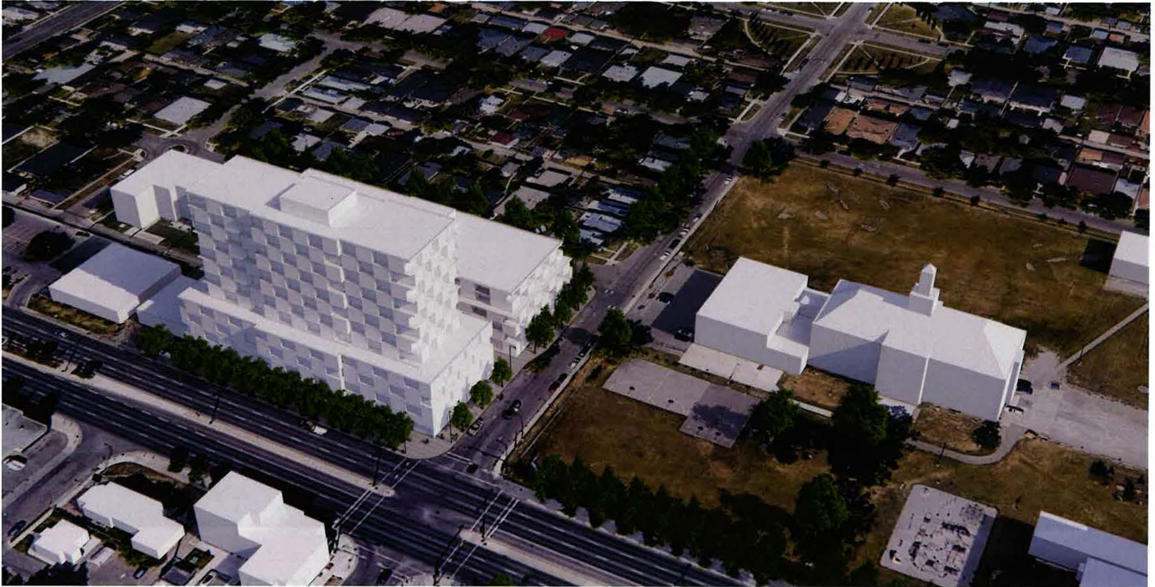
AERIAL VIEW FACING NW
