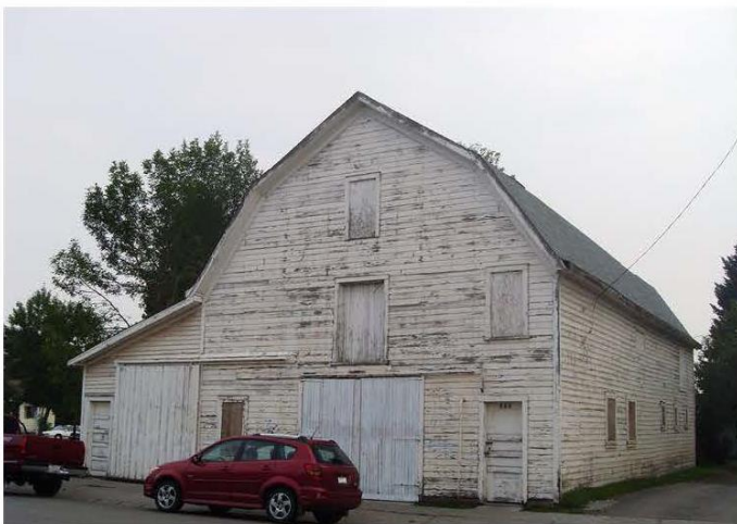
Stewart Livery Stable, Inglewood, photo credit City of Calgary, 2019
