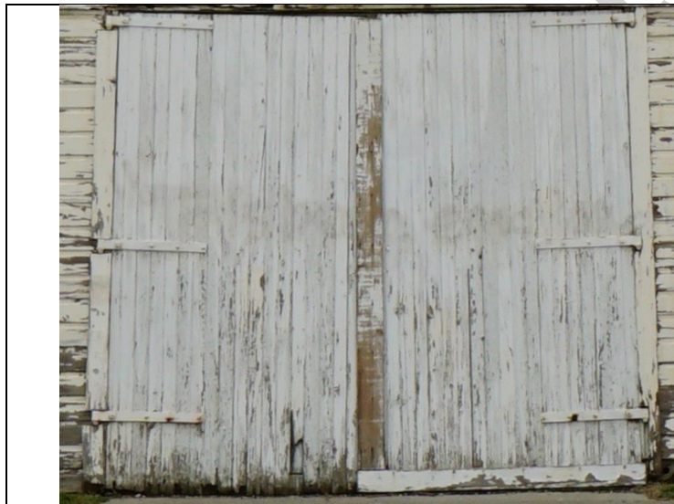
Image 2.2: Central wood double-doors and hardware
