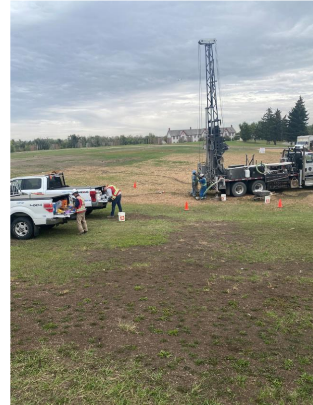
September 2023 Drilling for Geotechnical and Environmental Assessments
