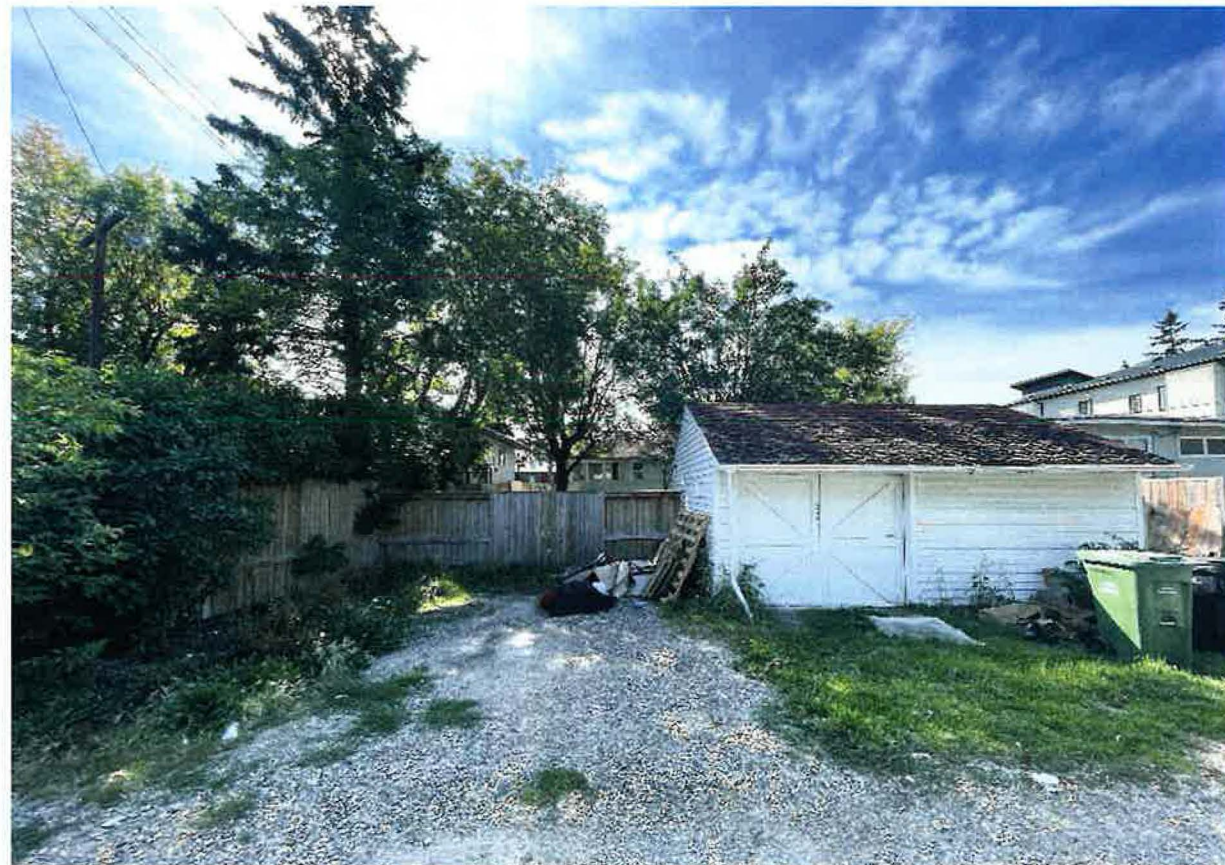
1212 - 20 Avenue NW from the lane
