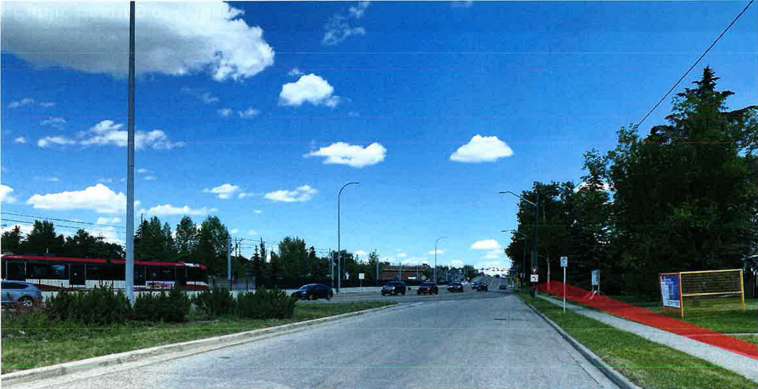
Looking East on 17 Ave SW
