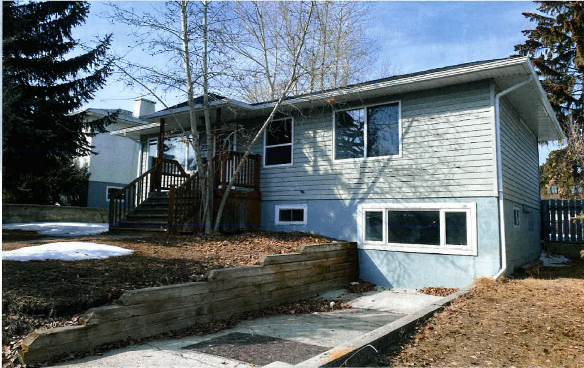
View from 26 Ave SW
