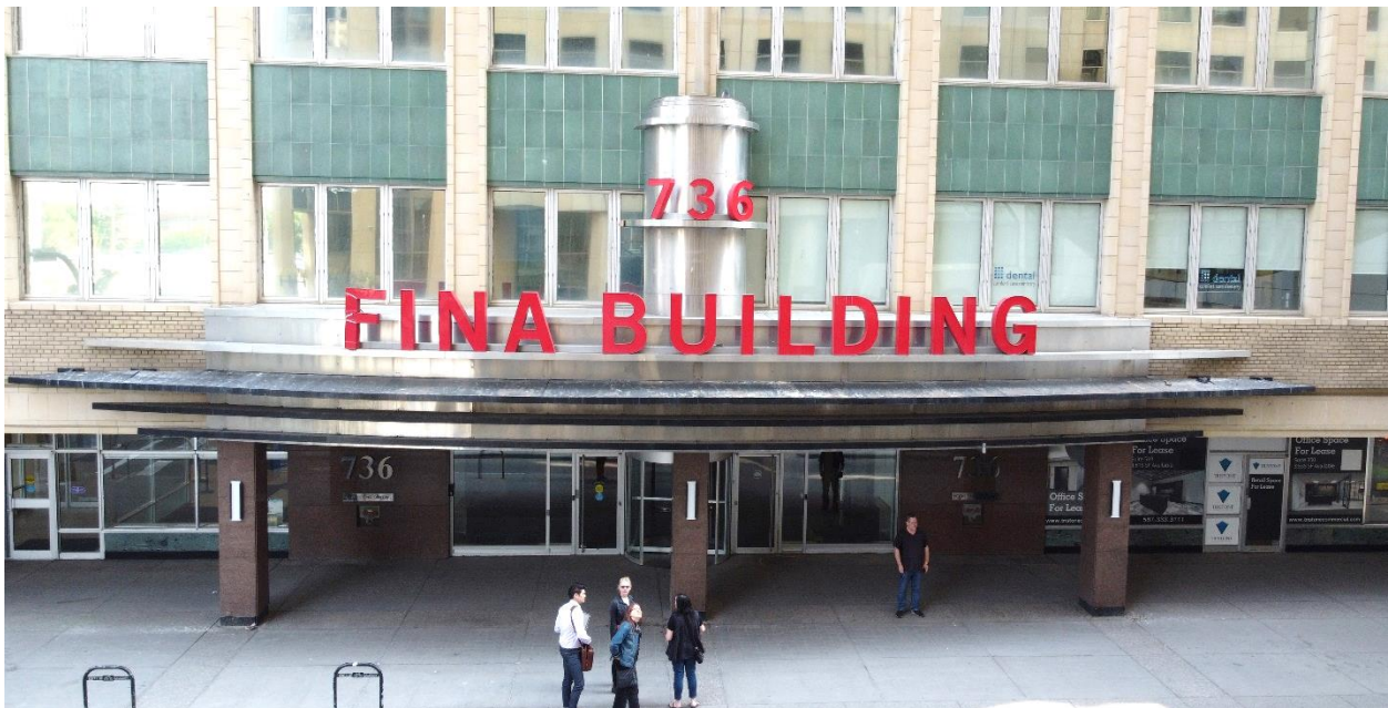
(Image 3.13: Ground level arcade formed between granite columns, recessed commercial storefronts, granite clad feature wall and lobby entrance)
