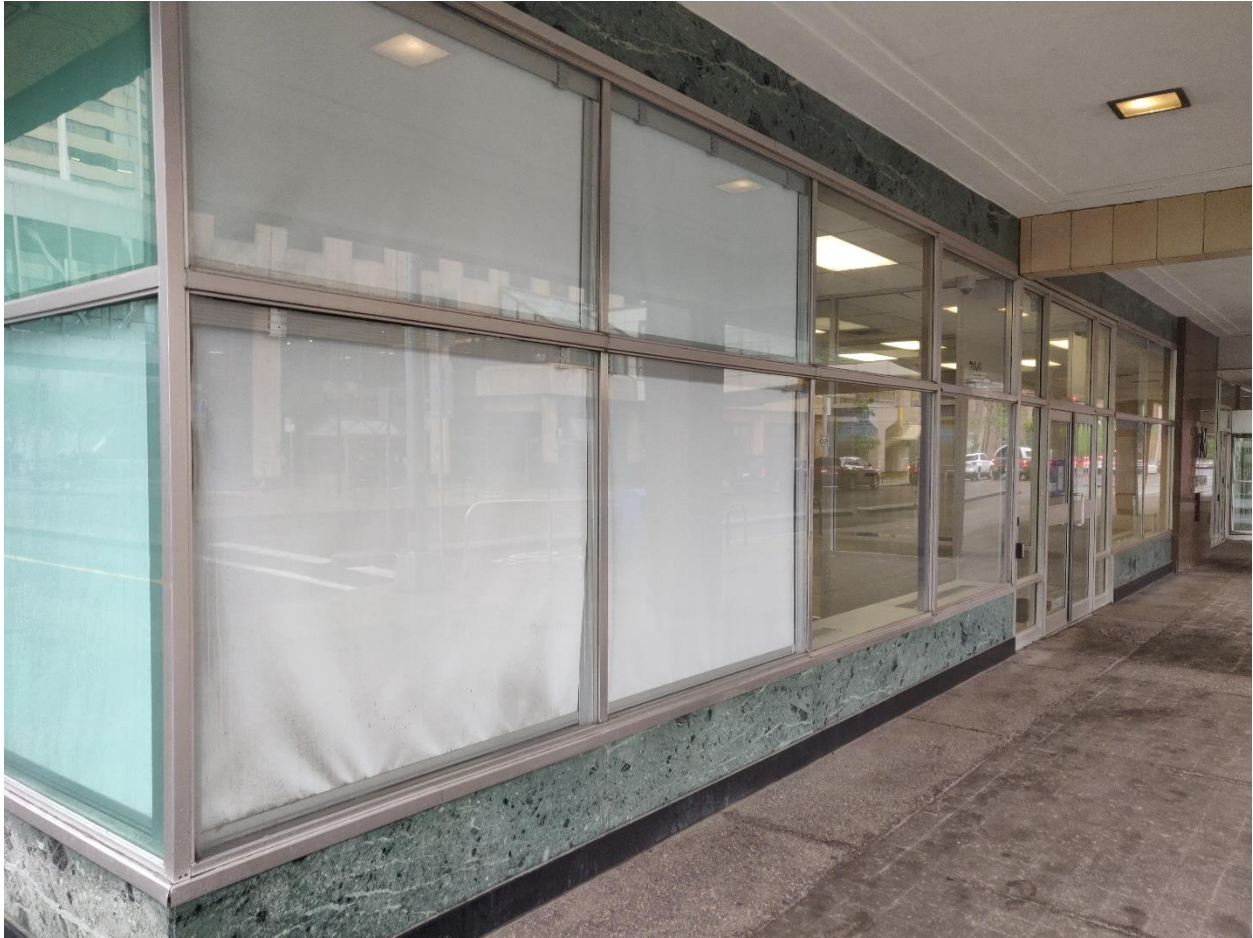
(Image 3.11: Glazed recessed display windows and commercial storefront with upper bands and bulkheads clad in green toned 'verde issorie' marble)
