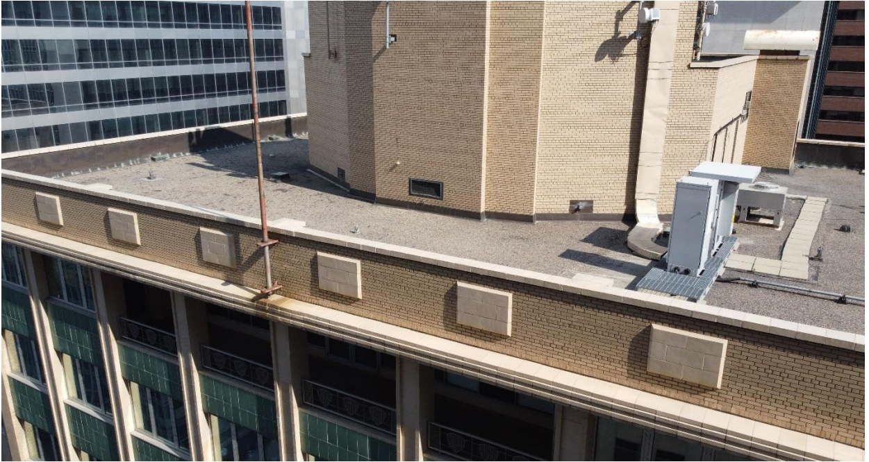
(Image 2.2: Parapet with glazed terra cotta coping, relief stone panels with projecting moulded canopy beneath – south façade)
