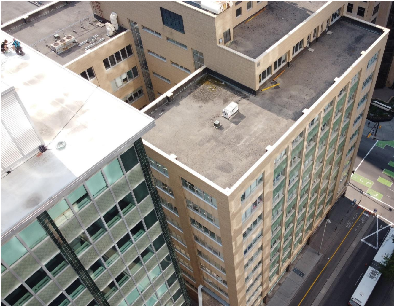
(Image 3.5: Aerial view of west façade and portions of north façade, north façade fenestration including repeating five-pane vertical window sash pattern, inset wall with evenly spaced multi pane narrow horizontal windows flanked by two vertical columns of multi pane windows, narrow aluminum tubular sashes, rooftop penthouse, elevator and mechanical structure)
