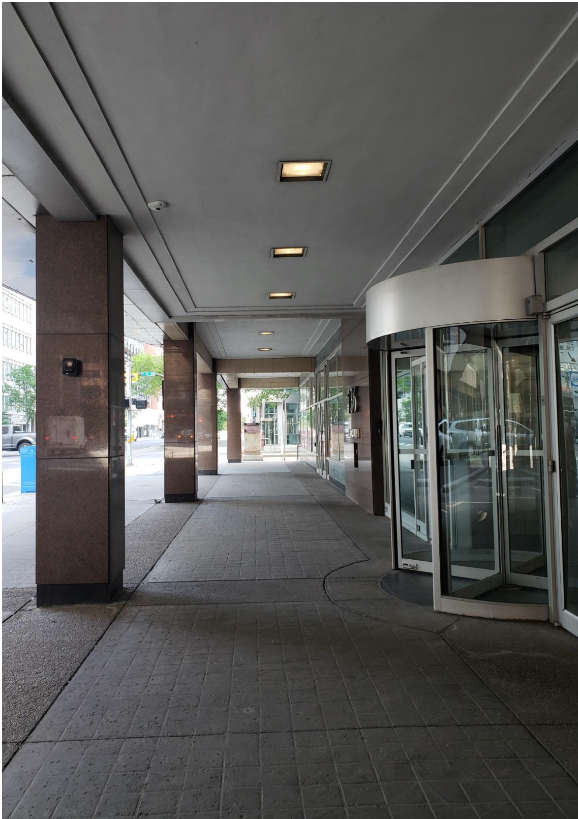
(Image 3.12: Ground level arcade formed between granite clad columns (on the left), commercial storefronts, granite clad feature wall and lobby entrance (on the right))
