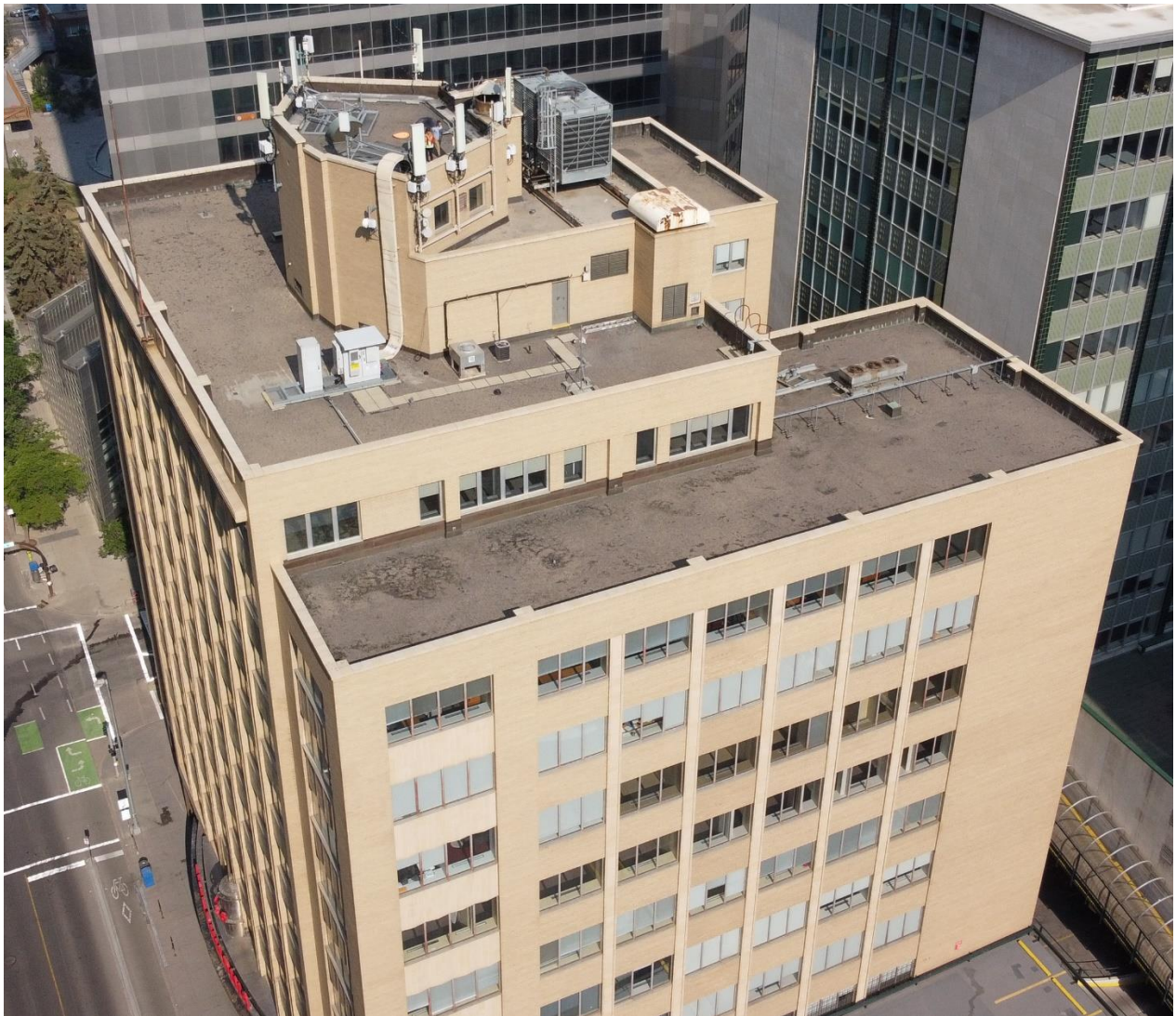
(Image 3.3: Aerial view of south and east façades, east façade fenestration including repeating three- and four-pane vertical window sash pattern, rooftop penthouse, elevator and mechanical structure)
