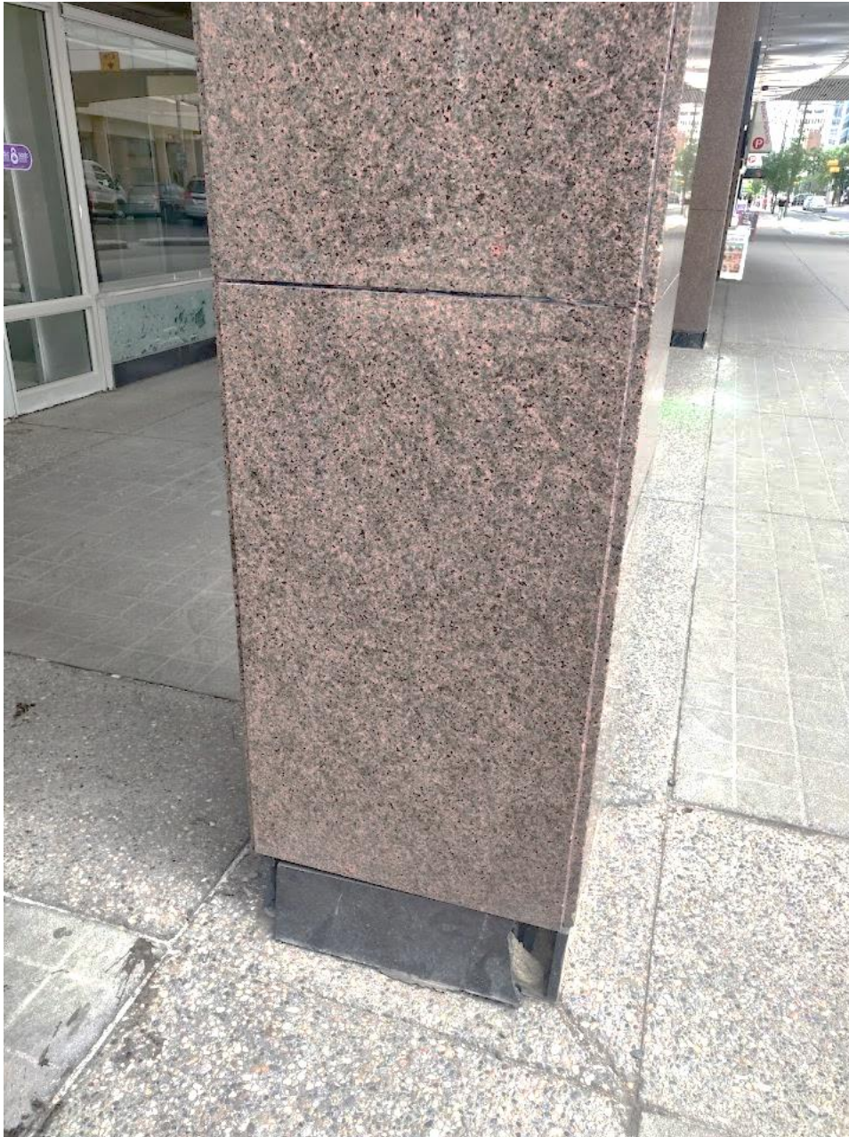
(Image 3.10: Detail view of a granite clad column)
