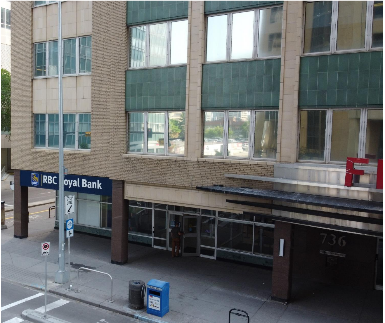
(Image 3.8: View of south façade's ground level arcade on southwest corner, showing granite clad columns, glazed moulded terra cotta signbands, and terra cotta sills on second storey, three- and four-pane vertical window sash pattern and narrow aluminum tubular sashes)
