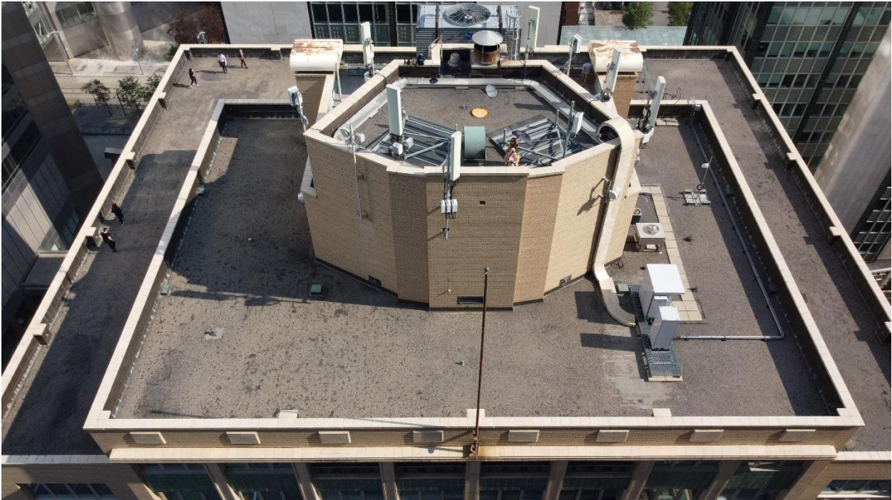
(Image 2.3: South-facing aerial view of roof showing stepped back rooftop penthouse, and buff-coloured brick clad elevator and mechanical structure finished with terra cotta coping)
