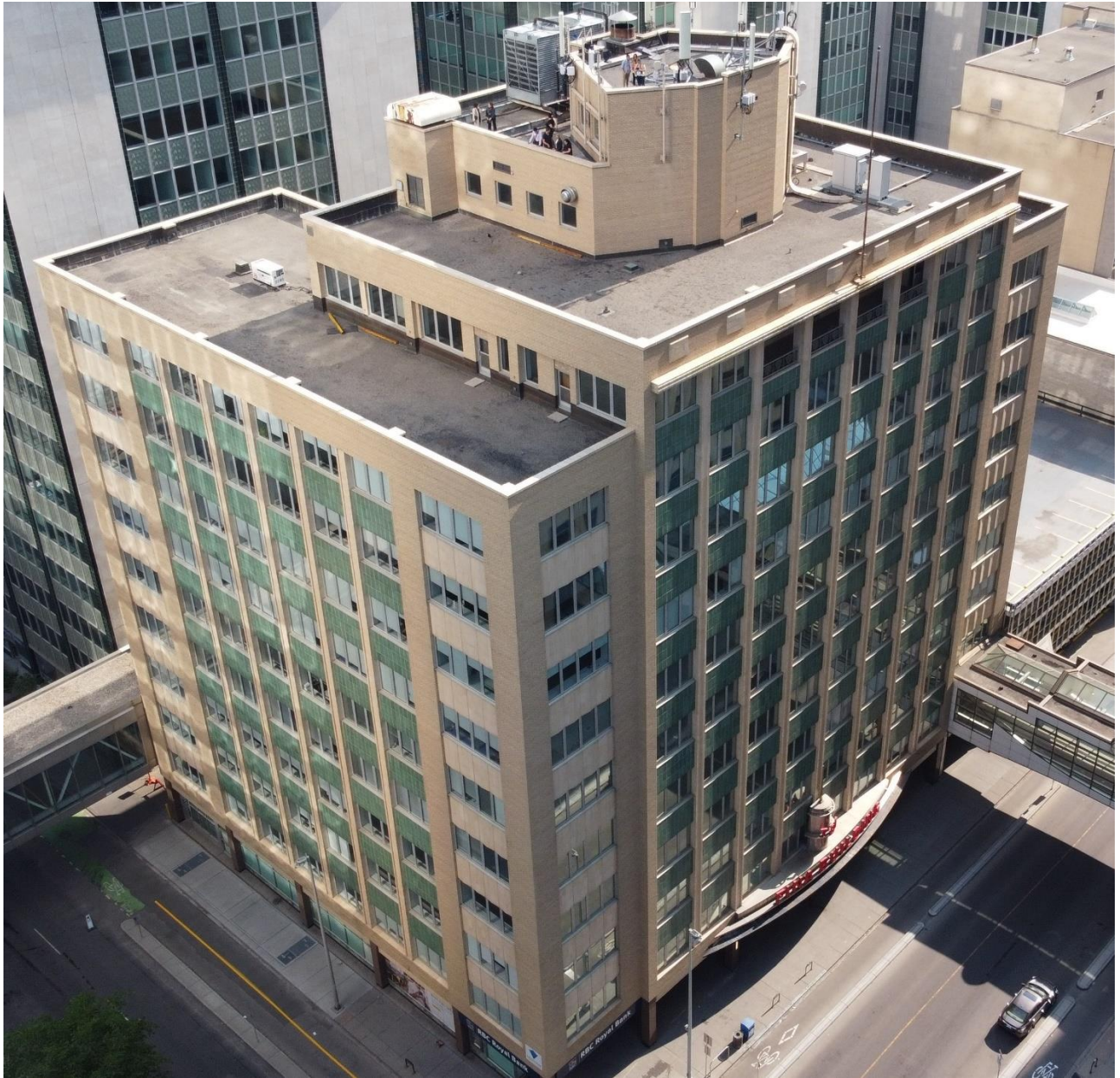
(Image 3.2: Aerial view of south and west façades, fenestration including repeating three- and four-pane vertical window sash pattern, rooftop penthouse, elevator and mechanical structure)
