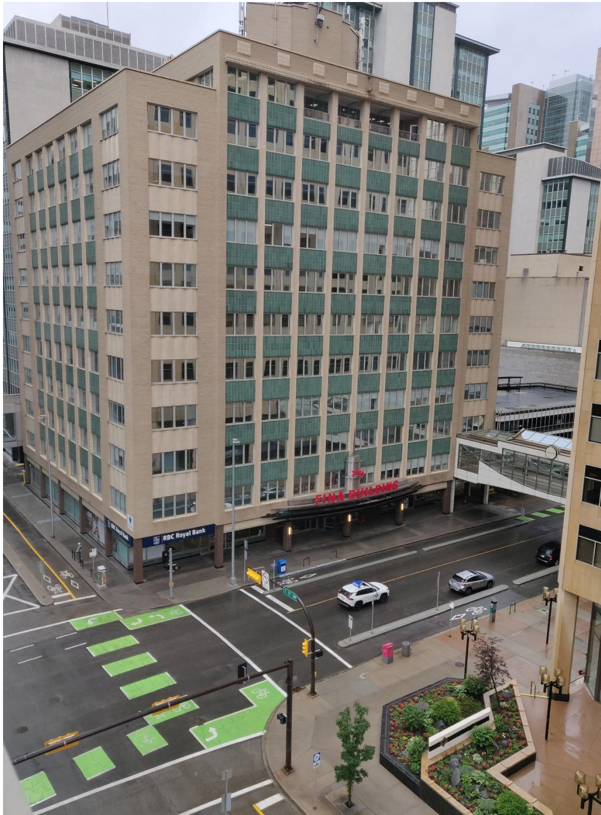
(Image 3.1: Oblique view of south façade – Petro-Fina building)
