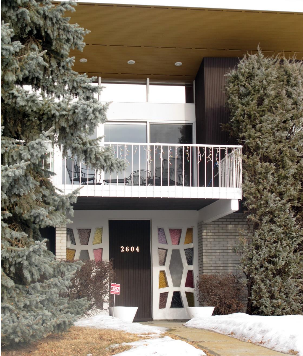
(Image 3.2: Detail of south façade, 2019 showing front entryway recessed under balcony supported by exposed beams and front door flanked by coloured-glass sidelights. Overhanging eaves, vented narrow wood slat soffits with pot lights also visible)
