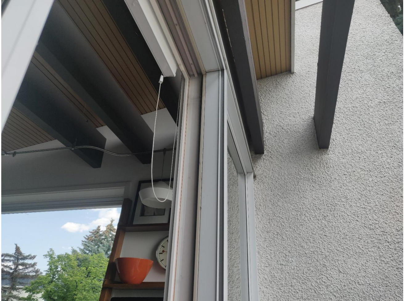
(Image 7.2: Exposed wooden beams, two of which are fully exterior and the other three interior, continuing through until ends are projecting on east facade)
