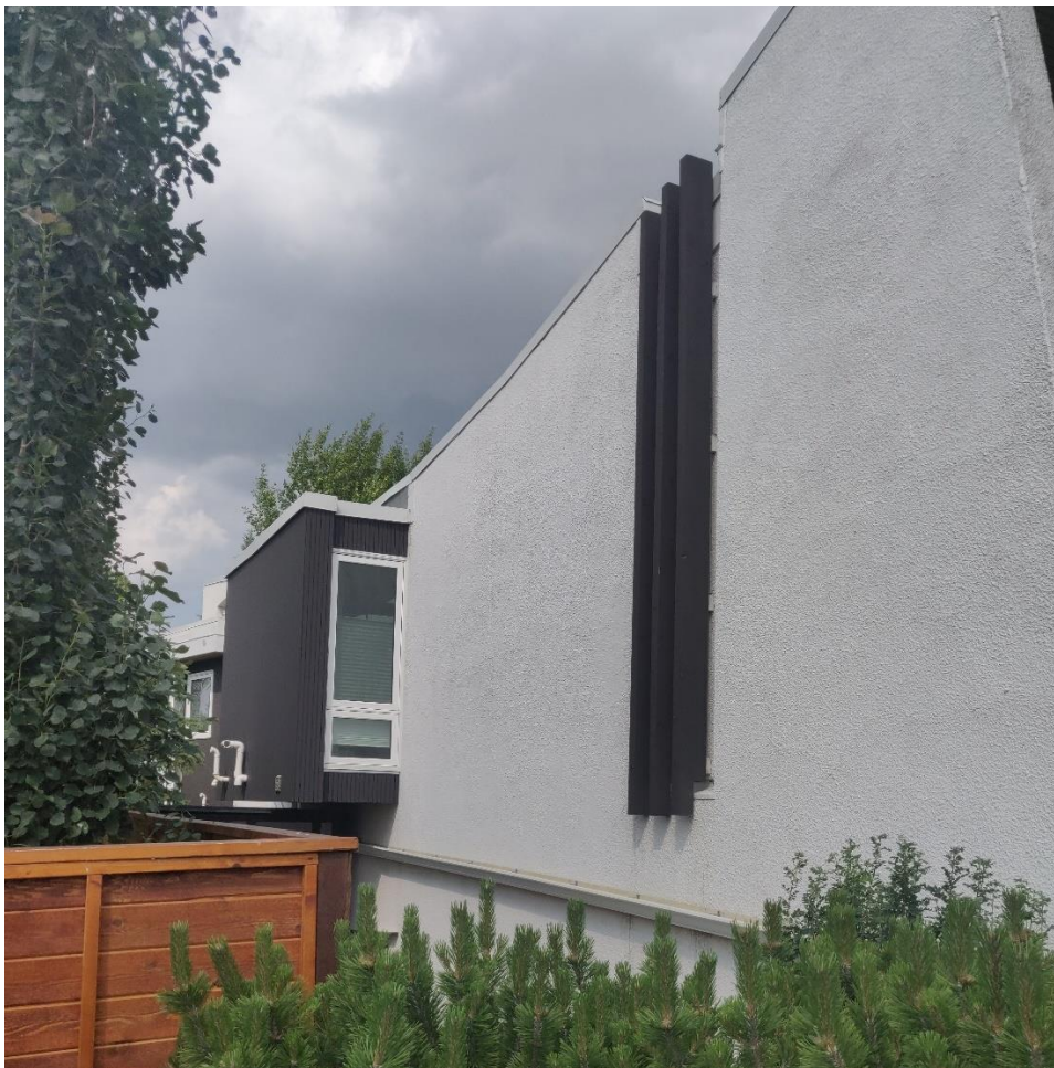
(Image 5.1: Oblique view of west façade showing tapered walls, cantilevered bump-out with vertical window opening, recessed wall with three projecting vertically-oriented wood slats)
