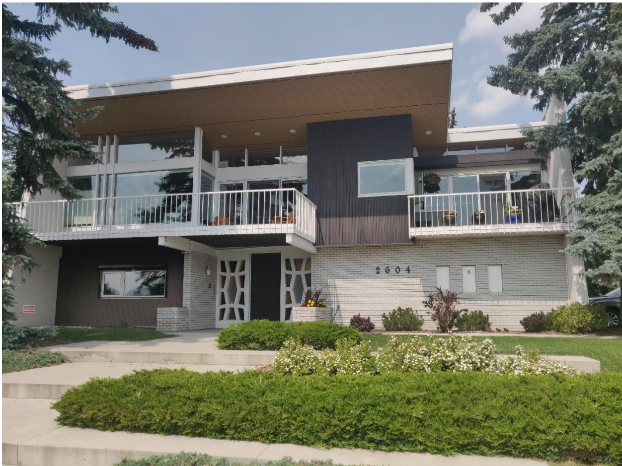
(Image 3.1: South façade of the Kalbfleisch Residence, facing Toronto Crescent NW)
