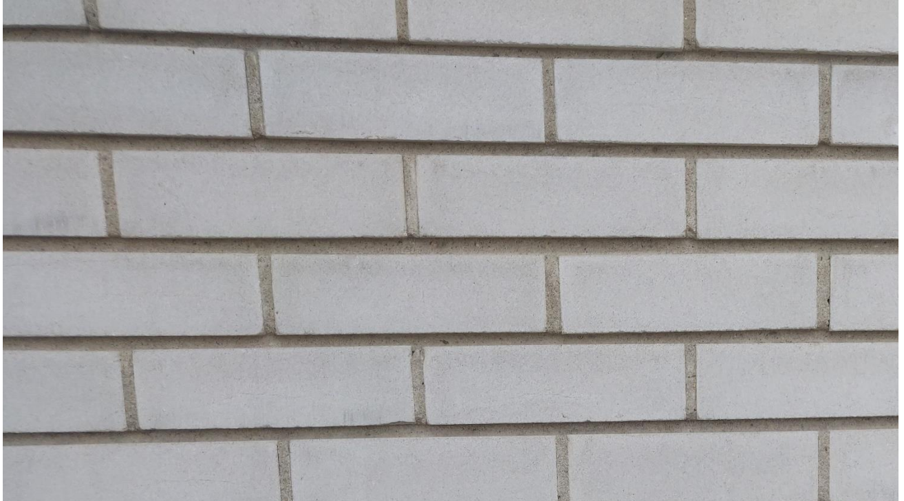
(Image 3.4: Detail of cream-coloured brick with horizontally-recessed and vertically-flush mortar)
