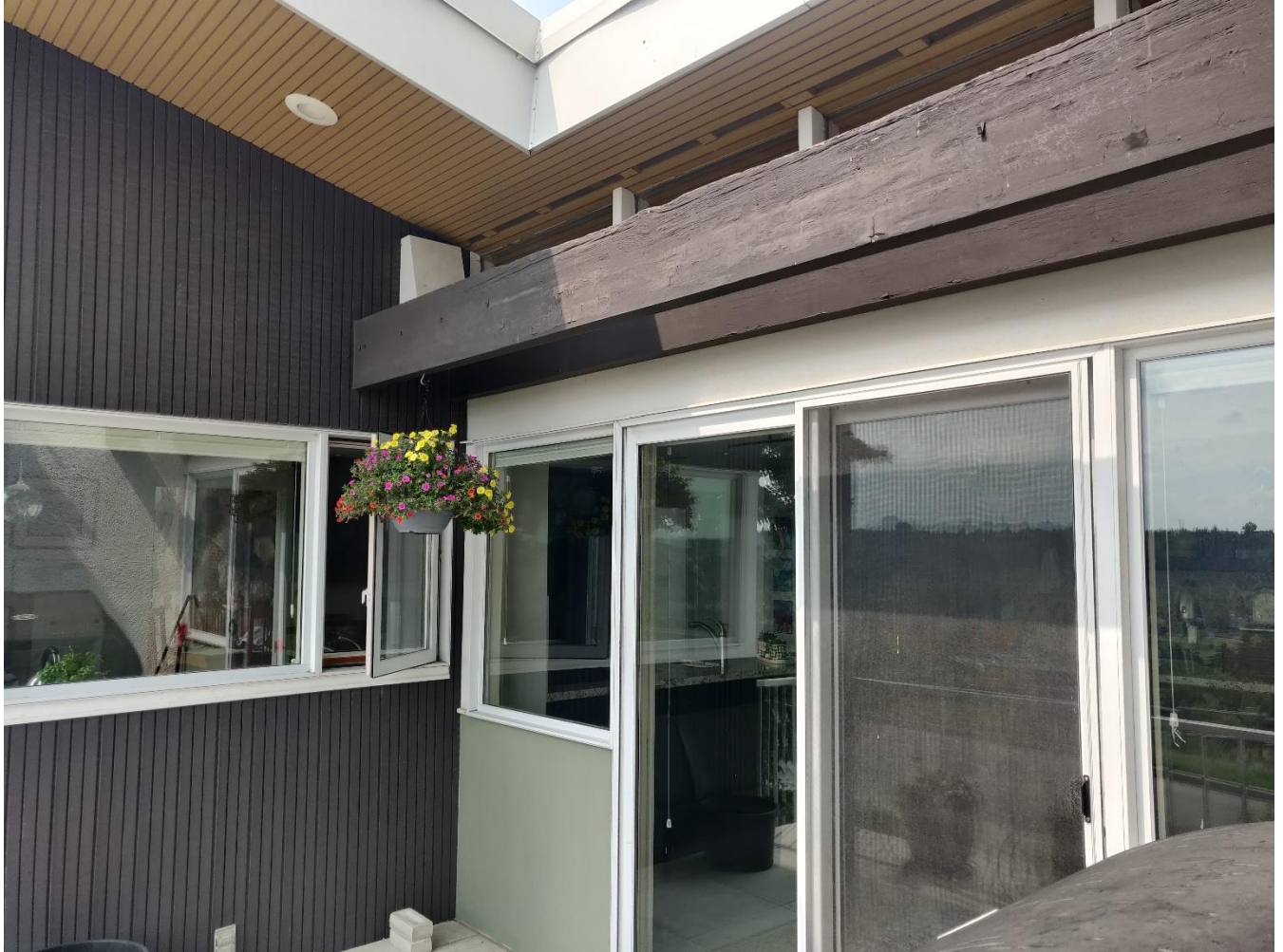
(Image 3.3: Detail of east-side balcony showing vented narrow wood slat soffits with pot light, exposed wooden beams, clerestory window and sash pattern, vertically-oriented narrow wood siding)
