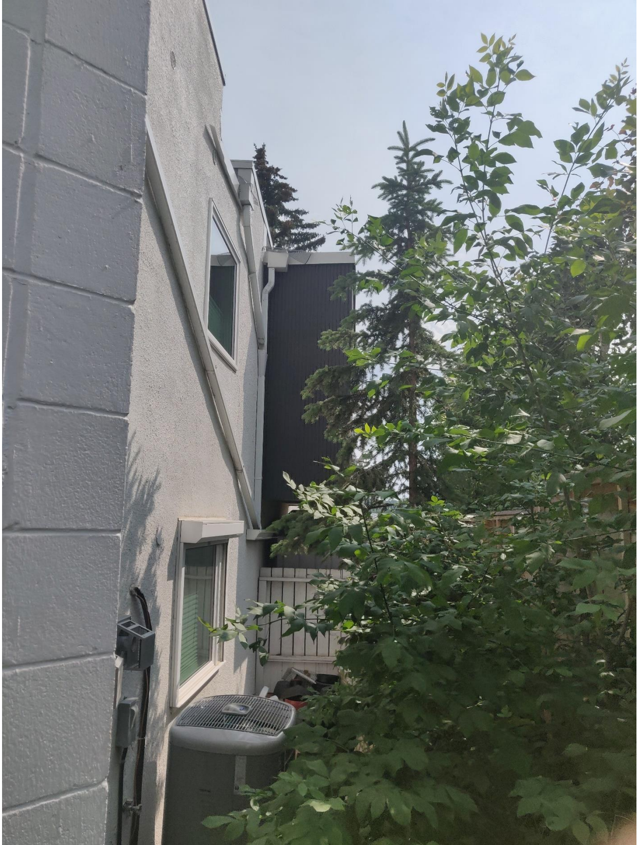
(Image 5.2: Oblique view of west façade showing the cantilevered bump-out from the north-west corner)
