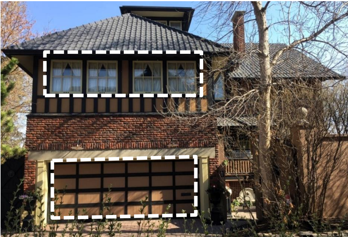
(Image 6.1: Northwest façade showing original garage extension, upper level veranda (originally sleeping porch now enclosed) Note: The areas demarked by the white dashed line (fenestration and the garage entrance) are not regulated)
