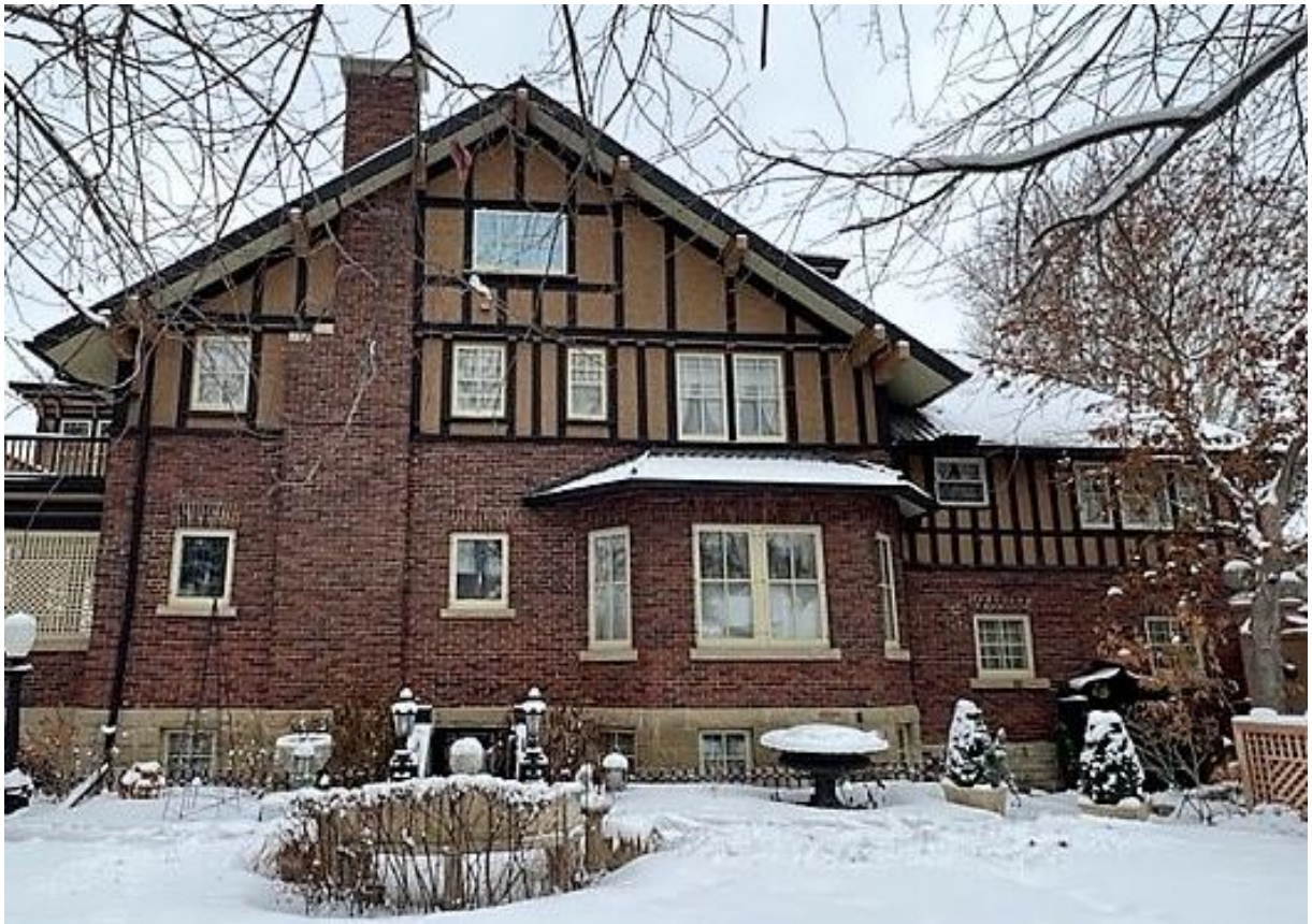
(Image 5.1: Northeast façade showing sandstone foundation; red brick cladding on the lower level; pebble-dash stucco and decorative wood half-timbering on the upper level wall and brick chimney, courtesy of R. McDonald)
