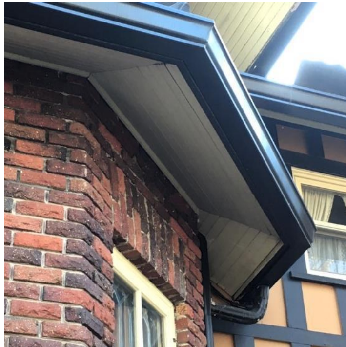
(Image 5.3: Detail of open, tongue-and-groove soffit above bay window)
