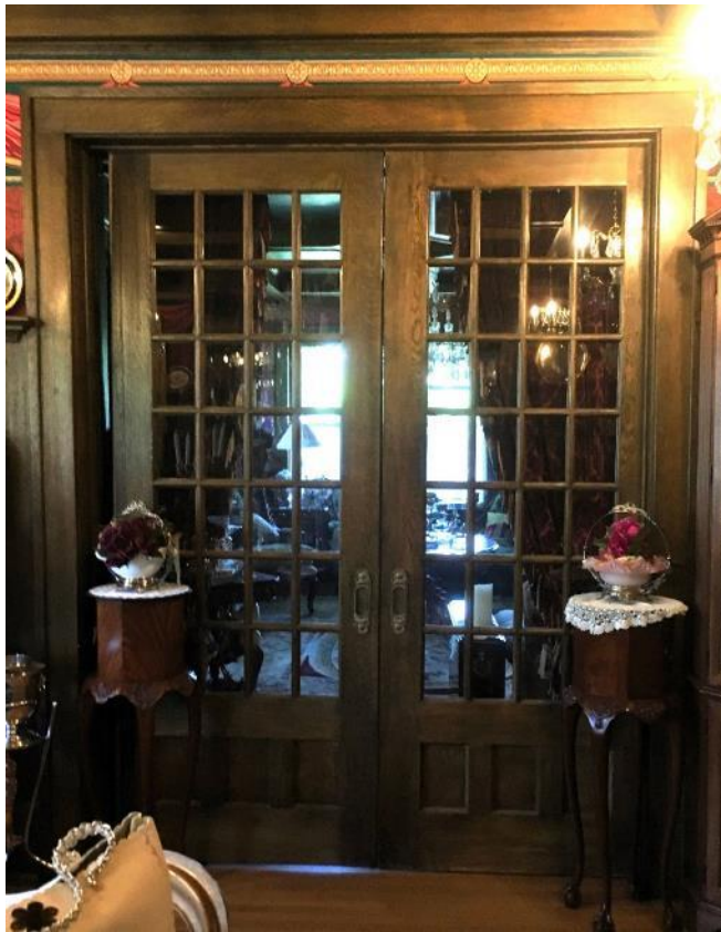
(Image 7.3: Oak wood glass and paneled pocket doors)
