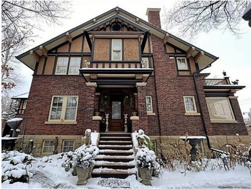
(Image 4.2: Southwest façade showing deep, open eaves; projecting purlins; exposed rafter tails, image courtesy of R. McDonald)
