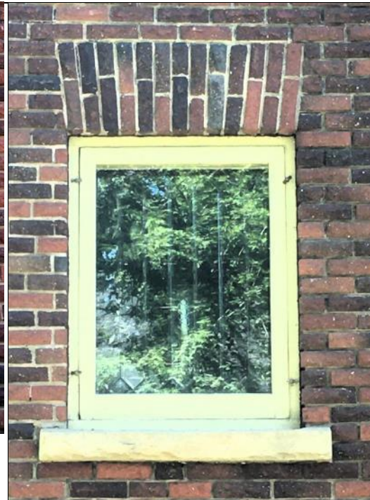
Image 5.5: Example of original fenestration, a fixed, multi-pane, beveled, leaded glass window. Note: Storm window in place over window.
