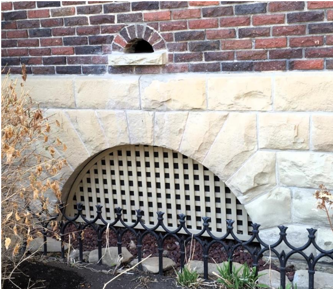
(Image 3.2: Example of sandstone foundation with radiating voussoir; verandah drainage opening with semi-circular arch and sandstone sill)
