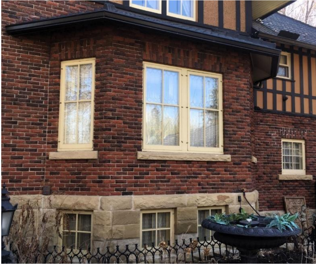
(Image 5.2: Detail of canted bay window. Note: Storm windows in place over windows.)
