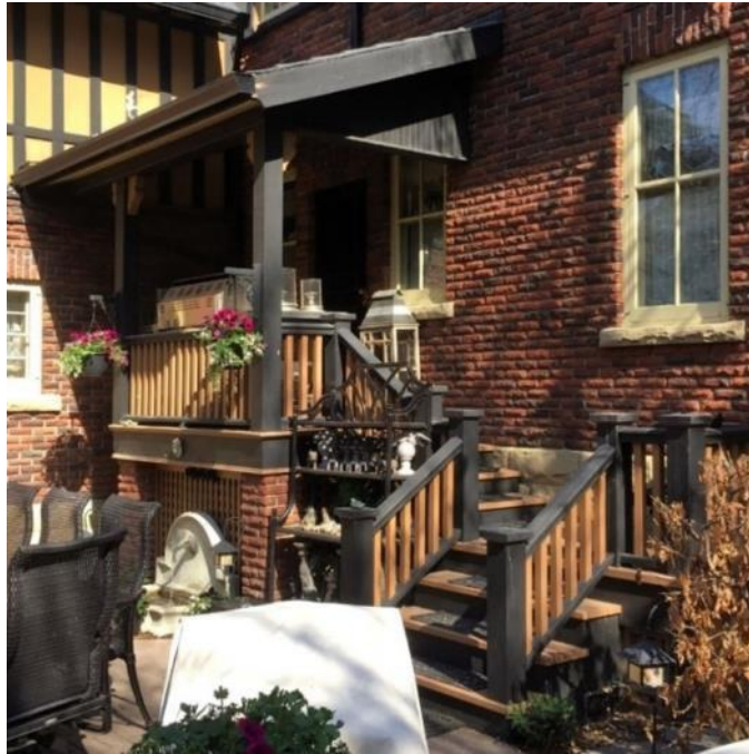
(Image 6.4: Detail of porch, shed roof, wood hand rail, posts, balustrade and brick piers)
