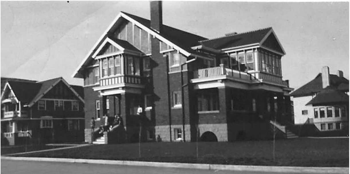
(Image 4.1: Historic oblique image of southwest façade prior to the southwest sunroom and attic fenestration changes)
