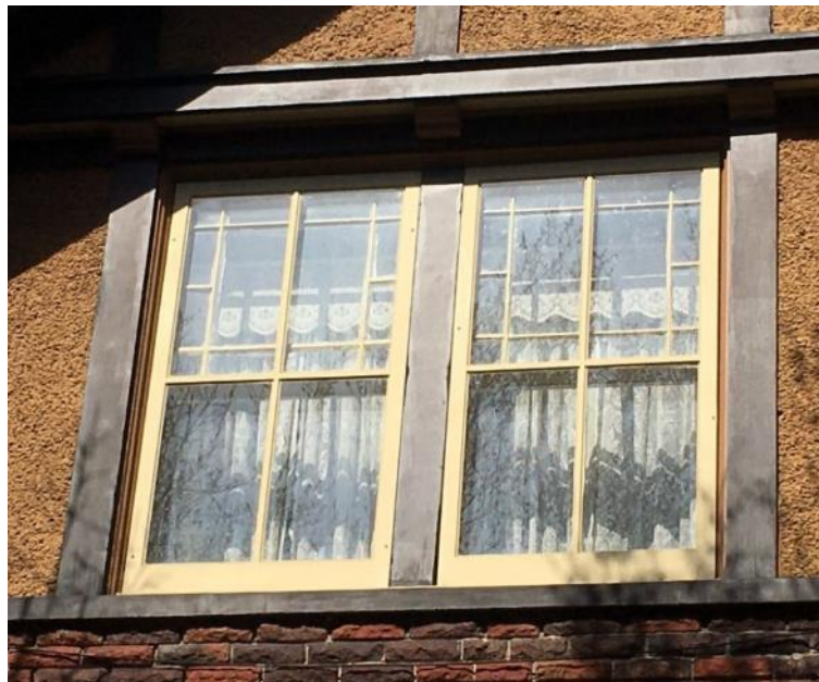
(Image 4.8: Detail of original fenestration, a paired assembly of multi-pane-glass-over-single pane windows, wood mullion and wood sill. Note: Storm windows in place over windows.)
