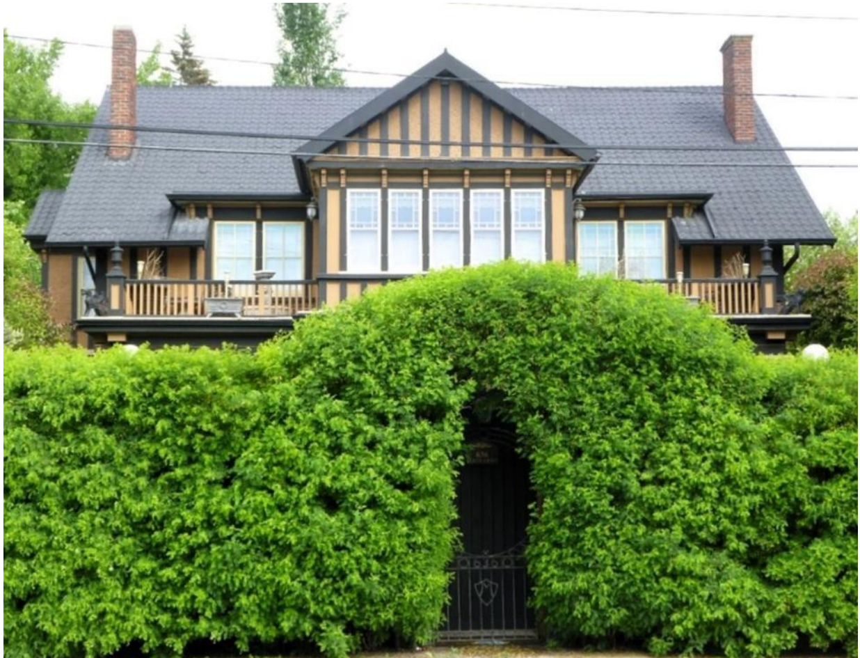
(Image 2.1: Southeast façade showing side-gabled roof and front-facing cross gable, shed roof wall dormers and balconies)
