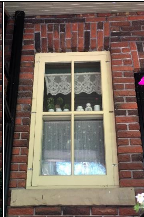
Image 6.6: Example of original fenestration, a one-over-one, single-hung window, jack brick arch header and sandstone sill. Note: Storm window in place over window.
