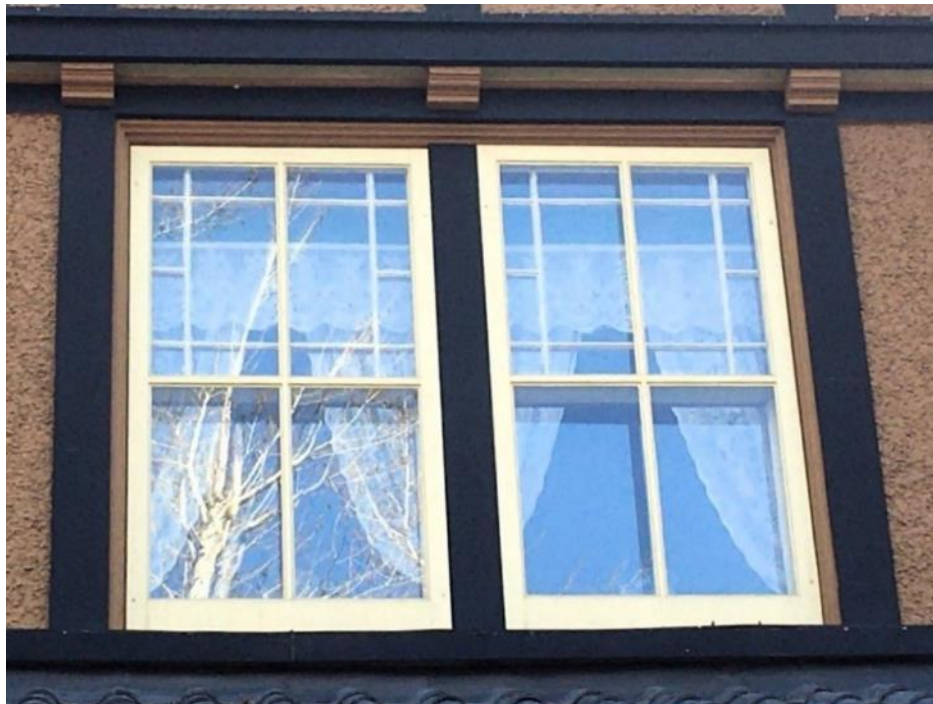
(Image 5.6: Example of original fenestration, a paired assembly of multi-pane-glass-over-single pane windows, wood mullion and wood sill. Note: Storm windows in place over windows)
