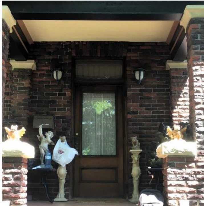
(Image 4.4: Detail of original side entryway oak wood door, multi-pane glass transom, jack brick arch header and brick pilasters with sandstone capitals)
