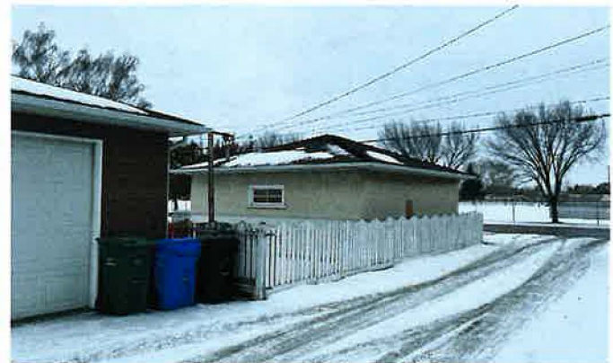
Looking Southwest from rear lane
