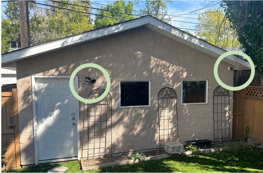
Separated motion-detection light and surveillance camera
