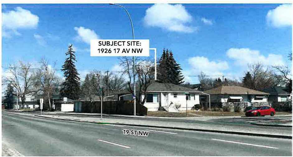
Looking Northeast from 19 ST NW
