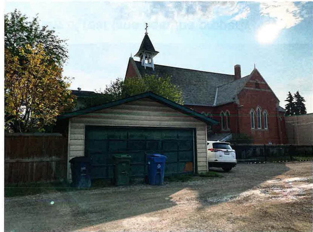
View from rear lane
