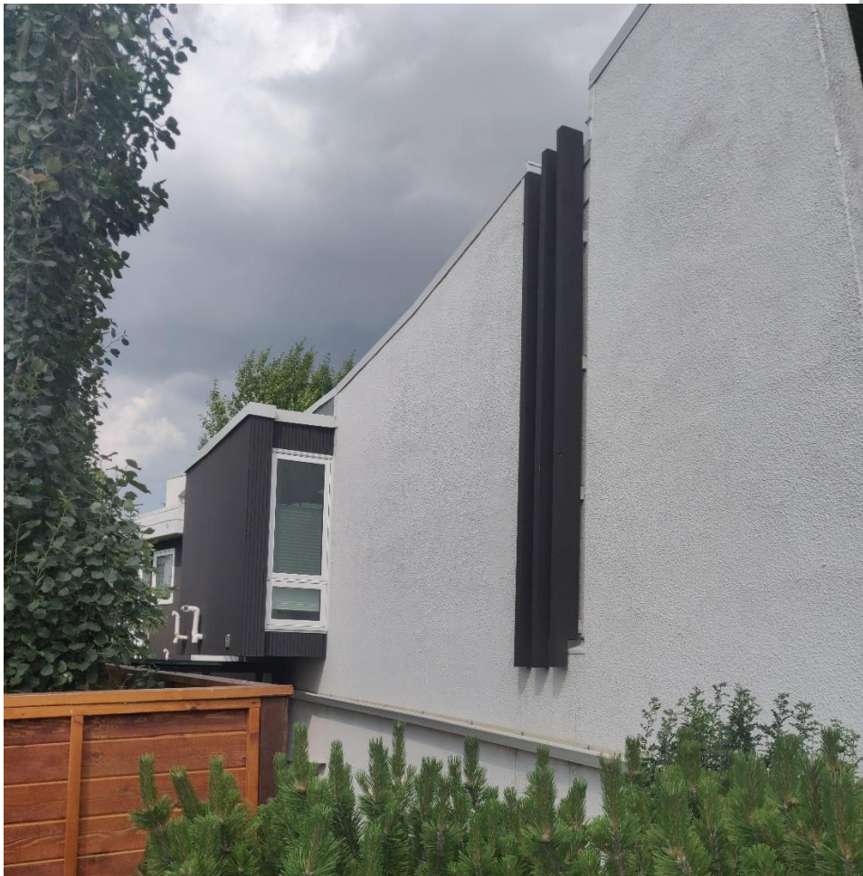
(Image 5.1: Oblique view of west façade showing tapered walls, cantilevered bump-out with vertical window opening, recessed wall with three projecting vertically-oriented wood slats)
