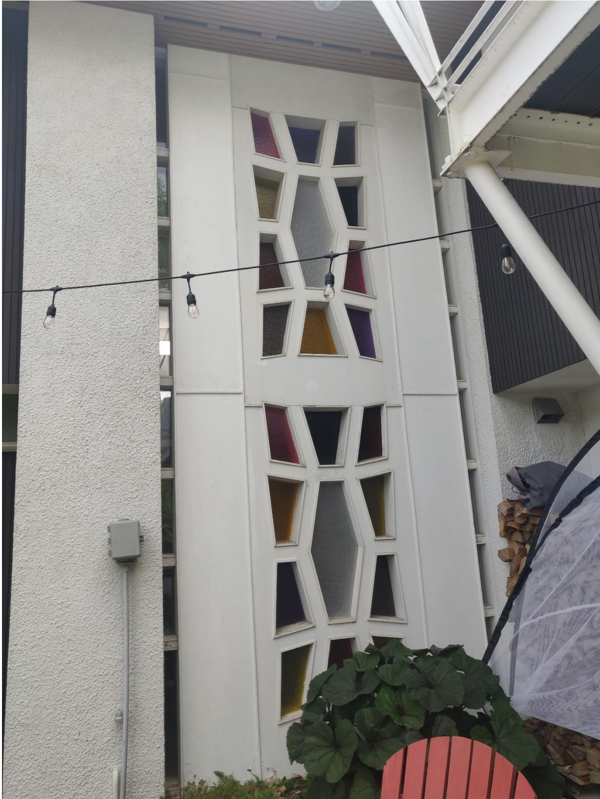
(Image 6.2: Photo of two-storey geometric coloured glass lights flanked by multi-pane sidelights and extant portions of stucco-clad bump-out. Vented narrow wood slat soffits and pot light.)
