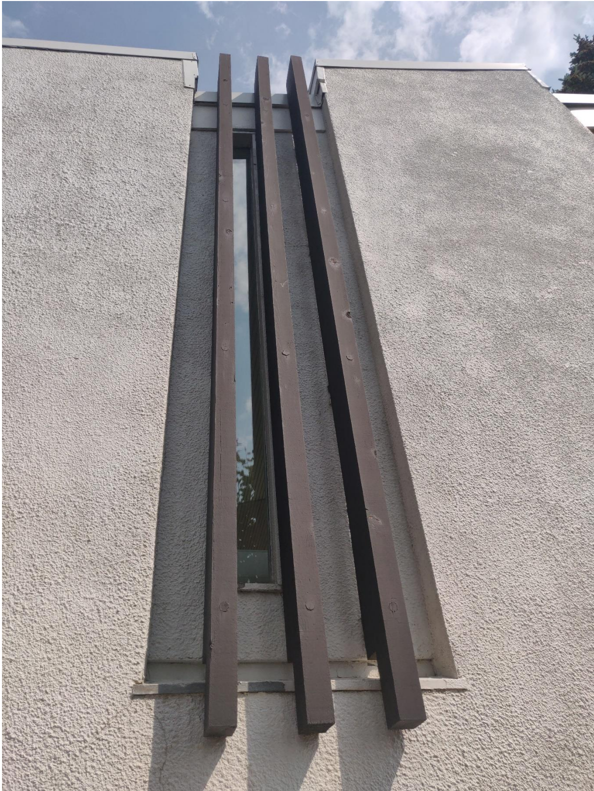
(Image 5.3: Recessed wall with tall narrow window slit and three projecting vertically-oriented wood slats)
