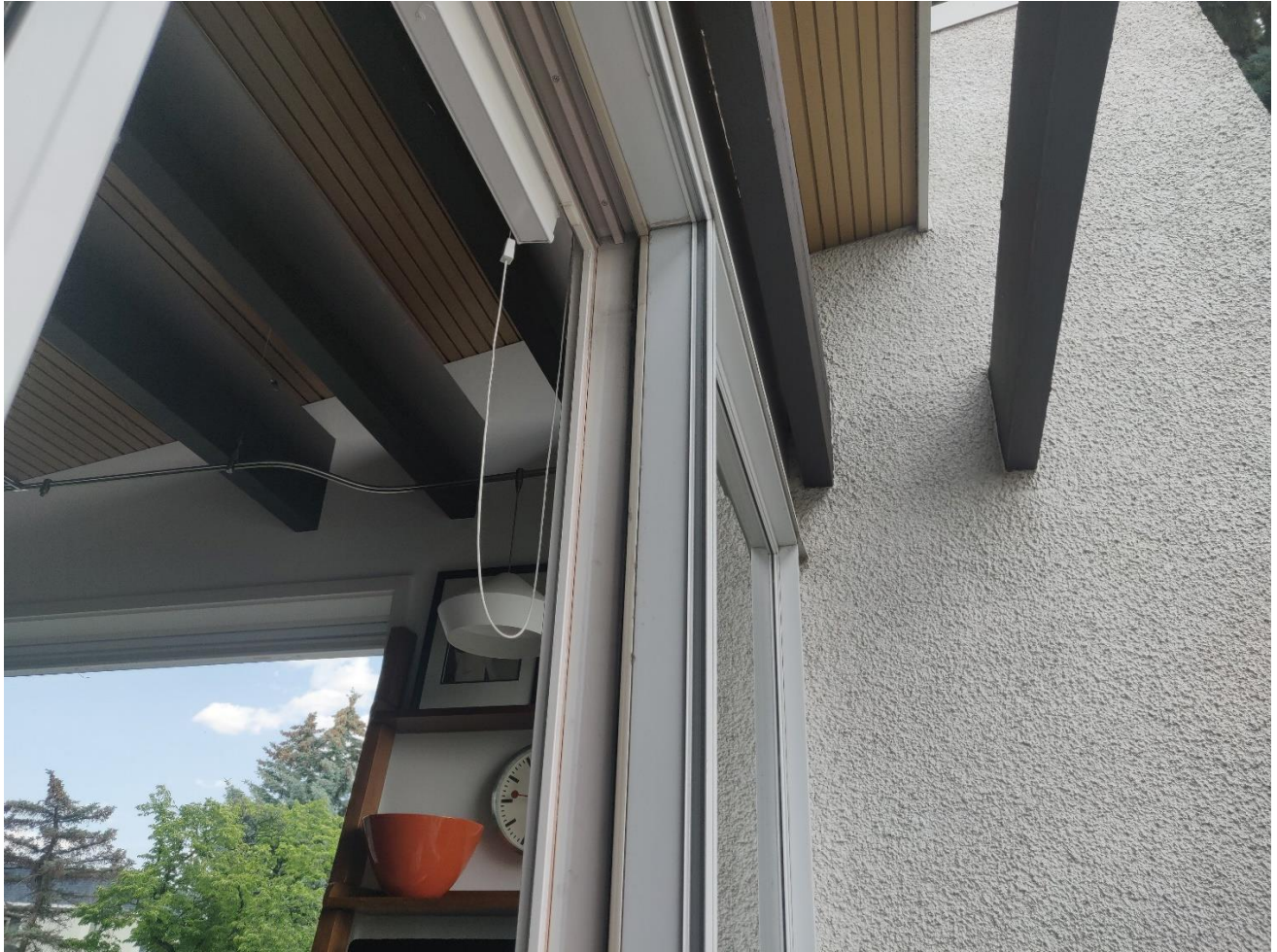
(Image 7.2: Exposed wooden beams, two of which are fully exterior and the other three interior, continuing through until ends are projecting on east facade)
