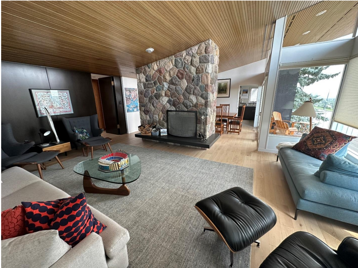
(Image 7.1: Split stone clad freestanding central fireplace with wraparound raised hearth extension. Detail of exterior east-west oriented narrow wood slat ceiling, continuing to the exterior. Photo Courtesy of Marc Poulin and Jean Rawling)
