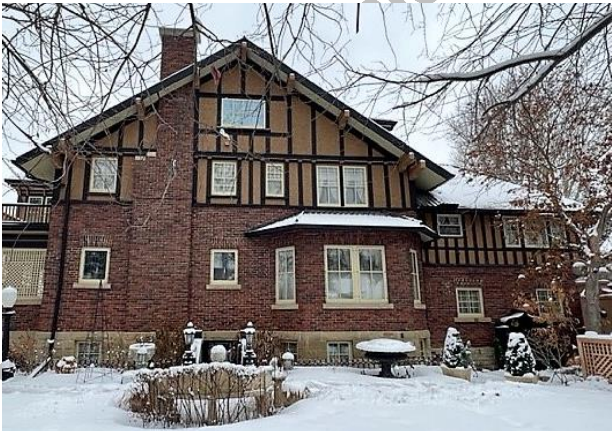
(Image 5.1: Northeast façade showing sandstone foundation; red brick cladding on the lower level; pebble-dash stucco and decorative wood half-timbering on the upper level wall and brick chimney, courtesy of R. McDonald)
