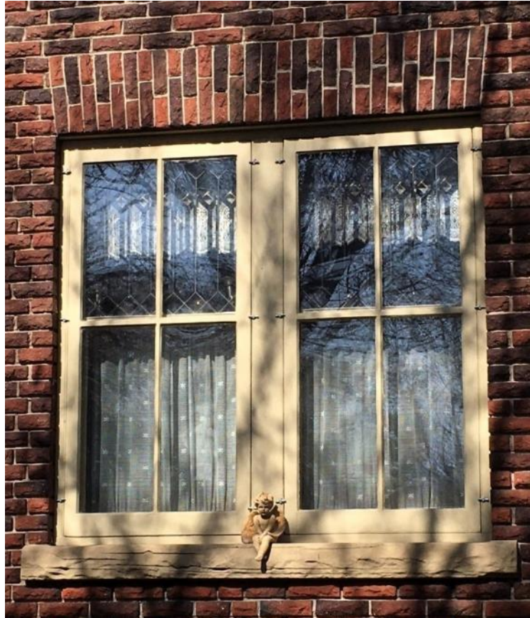
(Image 4.7: Detail of original fenestration, a paired assembly of multi-pane, beveled leaded glass-over-single pane windows, wood mullion, jack brick arch header and sandstone still. Note: Storm windows in place over windows.)
