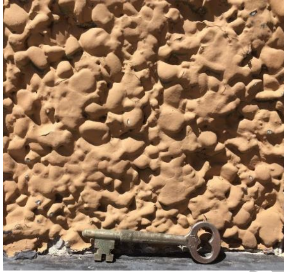
(Image 3.5: Detail of pebble-dash stucco comprised of small stones and applied 5 cm in depth)
