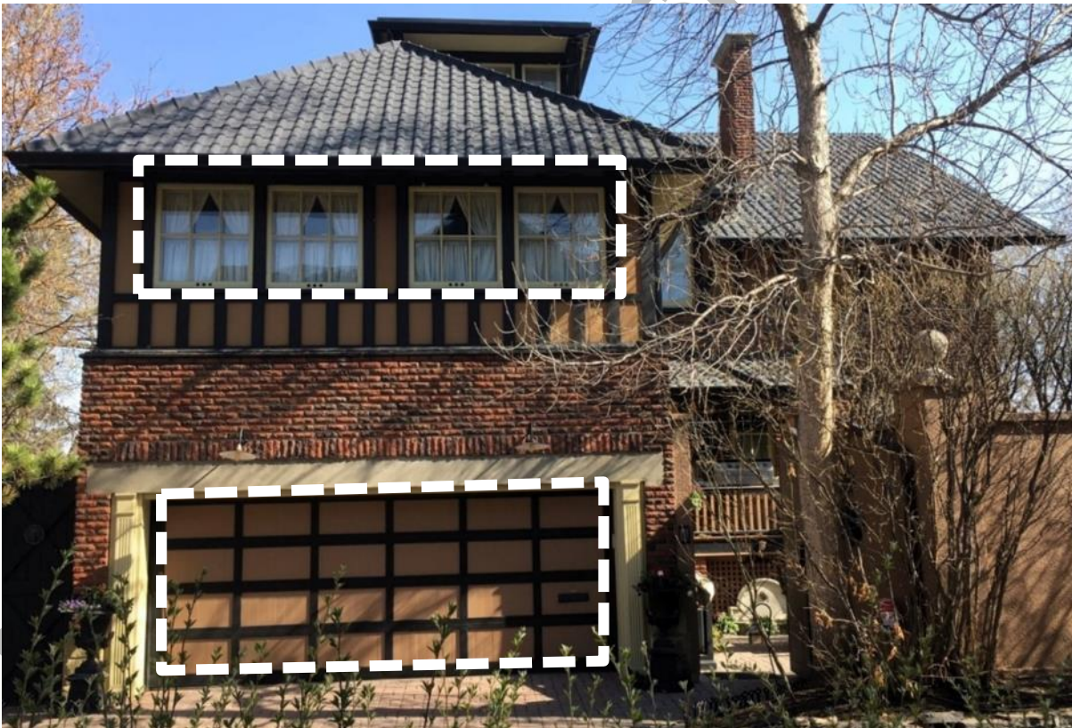
(Image 6.1: Northwest façade showing original garage extension, upper level veranda (originally sleeping porch now enclosed) Note: The areas demarked by the white dashed line (fenestration and the garage entrance) are not regulated)
