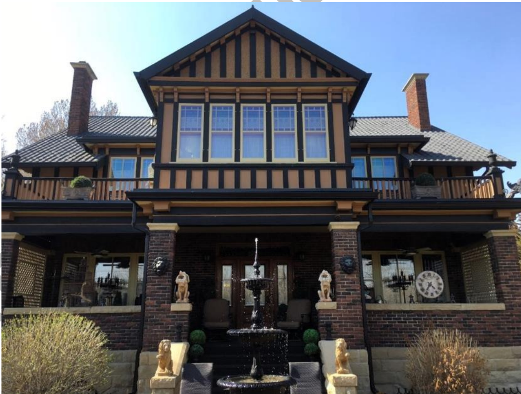
(Image 3.1: Southeast façade showing full width veranda and balconies above)
