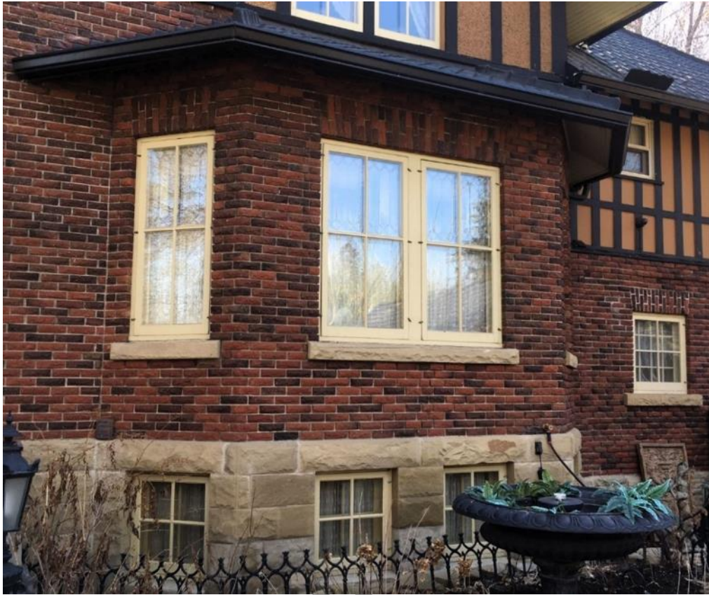
(Image 5.2: Detail of canted bay window. Note: Storm windows in place over windows.)
