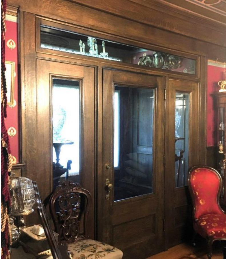
(Image 7.5: Oak wood vestibule with paneled and glass oak door, side lights and glass transom)
