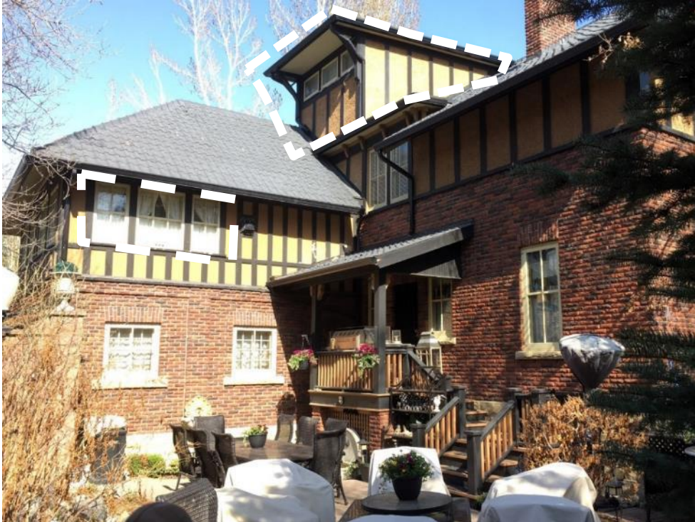
(Image 6.2: Oblique view of northwest façade. Note: The areas demarked by the white dashed line (upper shed roof dormer and upper level garage fenestration) are not regulated)
