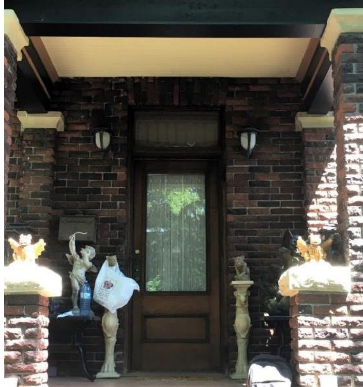
(Image 4.4: Detail of original side entryway oak wood door, multi-pane glass transom, jack brick arch header and brick pilasters with sandstone capitals)
