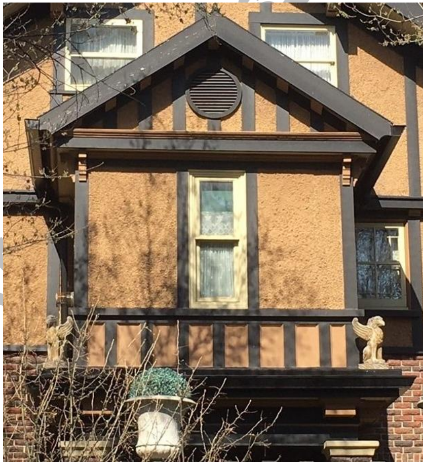
(Image 4.3: Detail of sunroom and paneled base)
