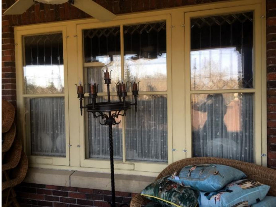
(Images 3.7: Example a triple window assembly, wood mullins, jack brick arch header and sandstone sill. Note: Storm windows in place over windows)
