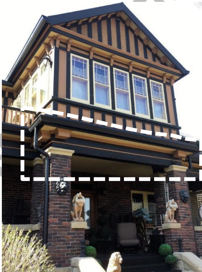
(Image 3.6: Southeast façade oblique image close up. The area demarked with white dashed lines details how the jettied sunroom rests on the projecting ends of the jetty joists above the paired sandstone capitals)
