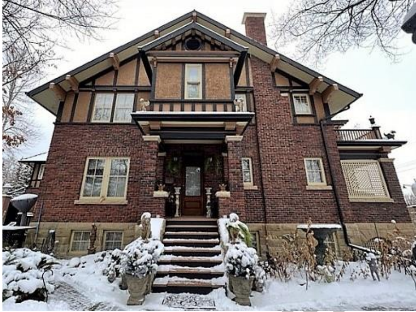
(Image 4.2: Southwest façade showing deep, open eaves; projecting purlins; exposed rafter tails, image courtesy of R. McDonald)
