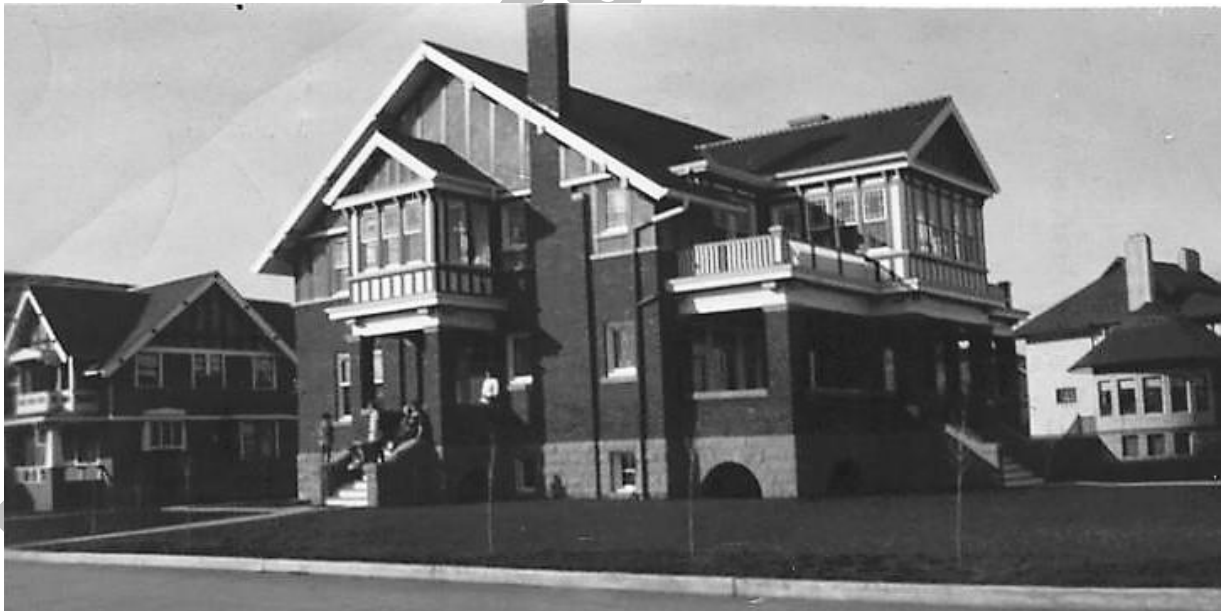
(Image 4.1: Historic oblique image of southwest façade prior to the southwest sunroom and attic fenestration changes)
