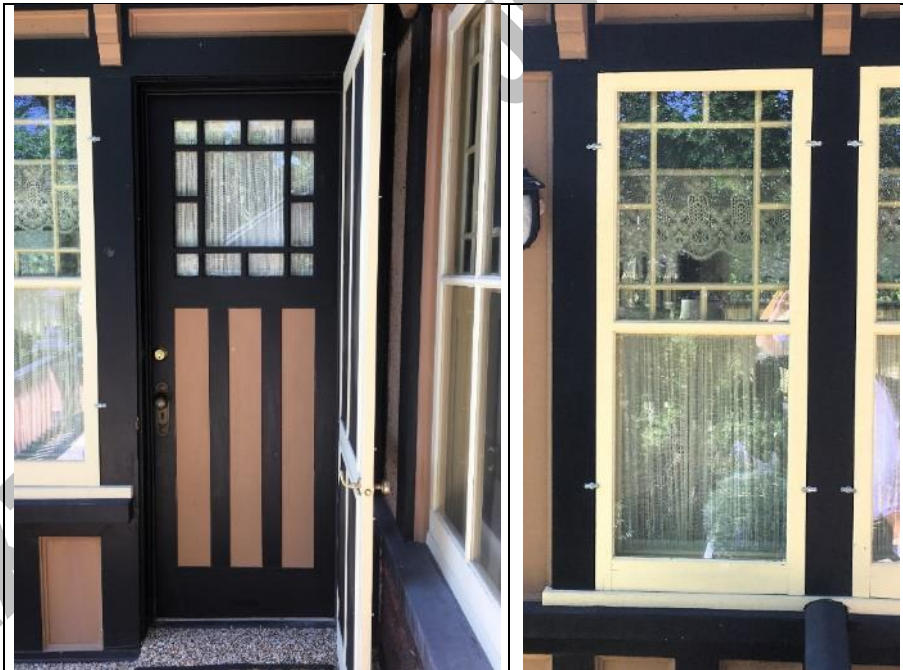
Image 3.8: Example of one of the multi-pane and three-panel French doors.
