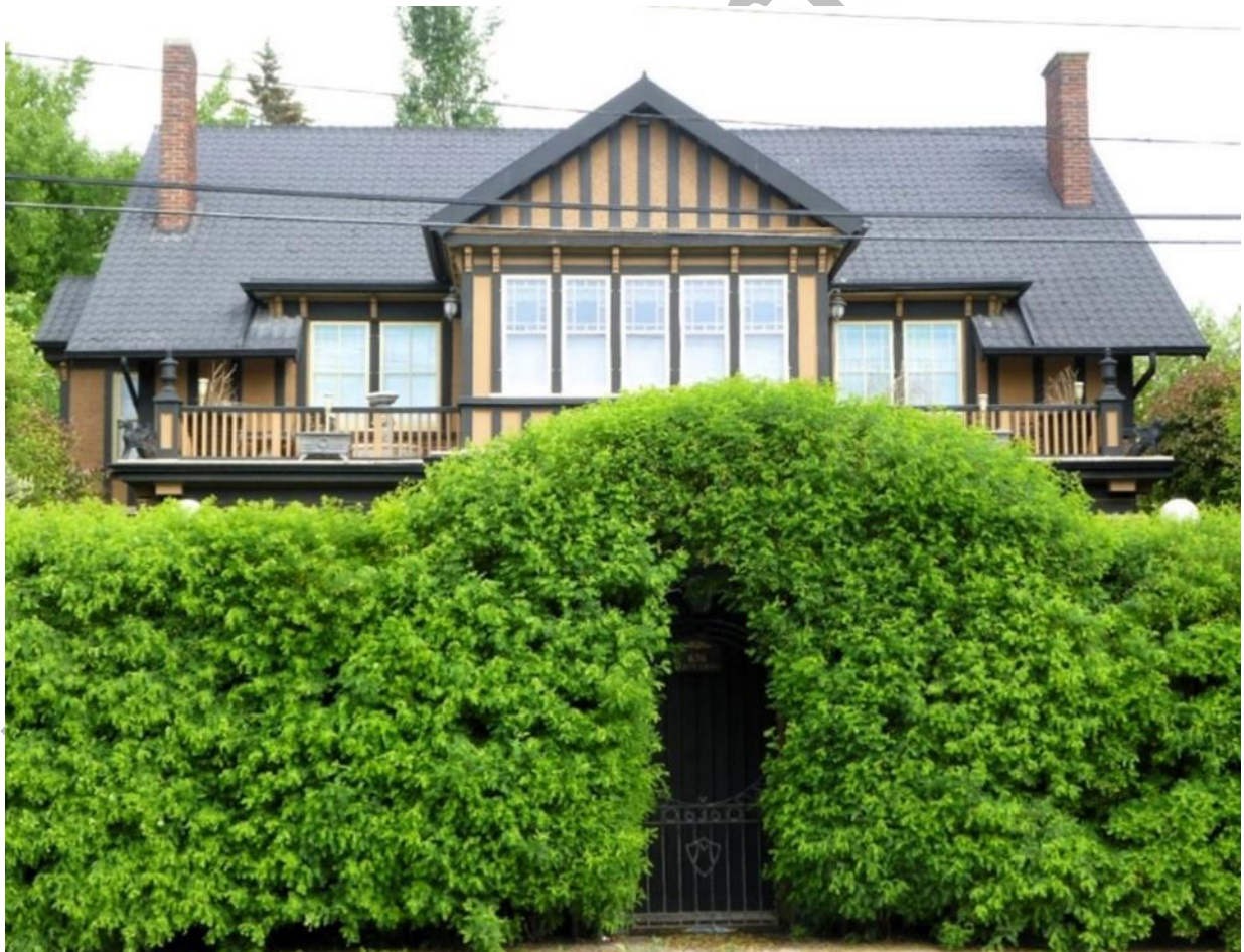
(Image 2.1: Southeast façade showing side-gabled roof and front-facing cross gable, shed roof wall dormers and balconies)
