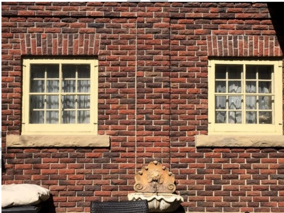
(Image 6.3: Detail of recessed brick panels on rear garage extension and original fenestration of multi-pane glass windows, jack arch brick headers and sandstone sills. Note: Storm windows in place over windows)
