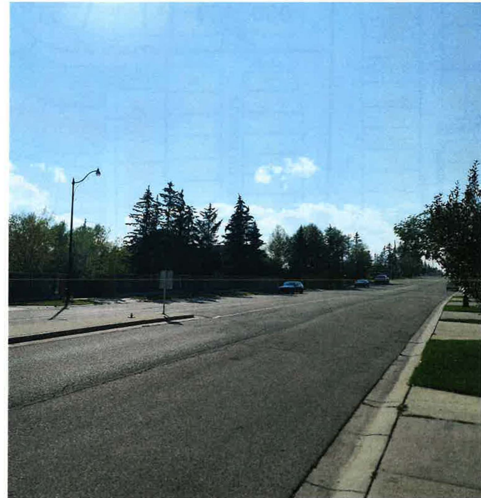
26 Avenue SW looking east
