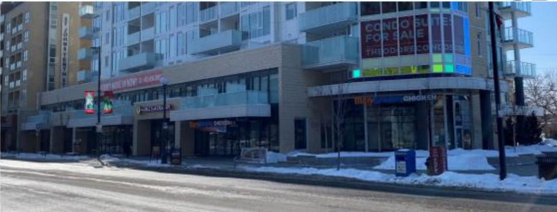
Figure 4: The existing Mary Brown's restaurant demonstrates how the Theodore's built form creates visually distinct store fronts with each commercial bay, despite being occupied by a single use.
