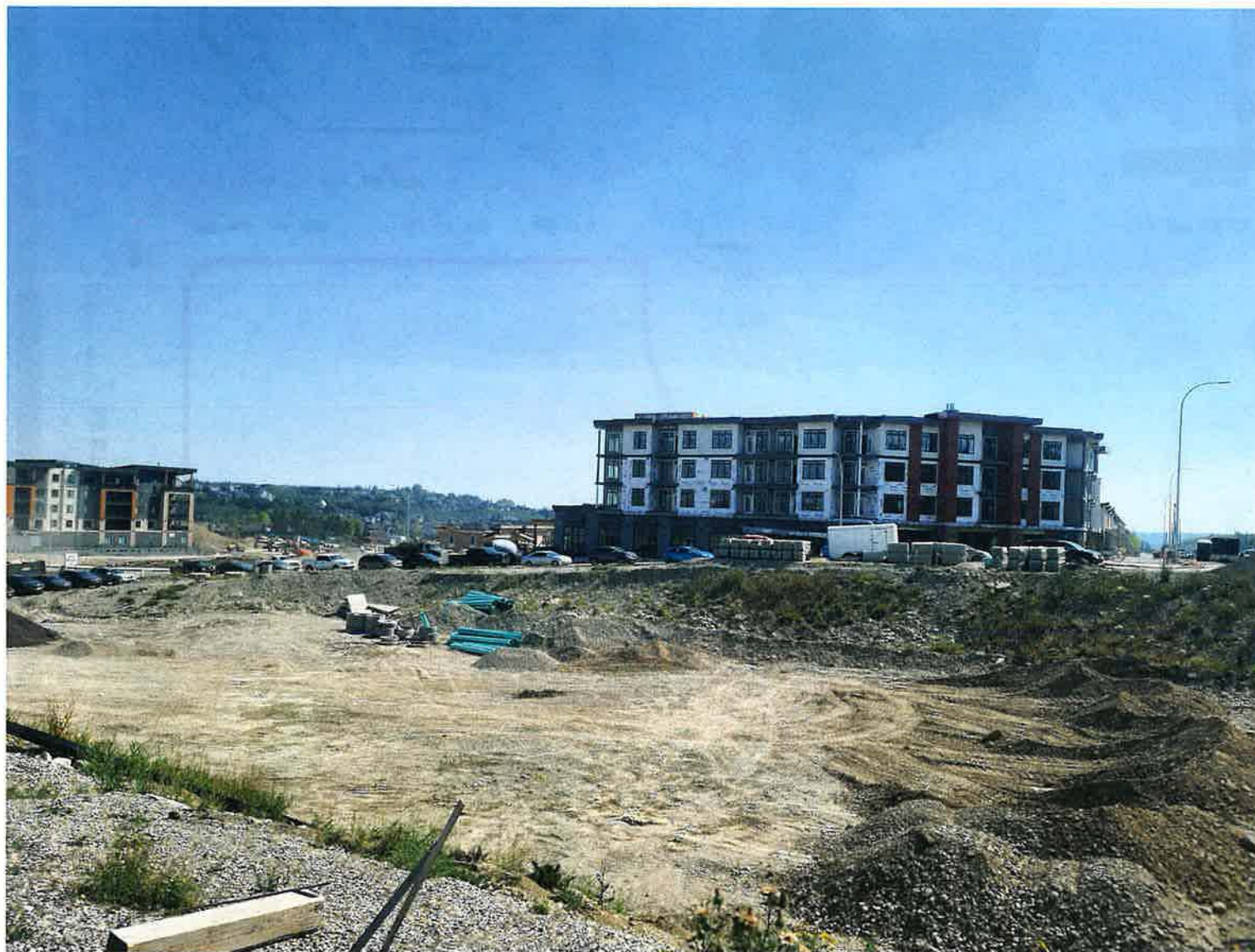
Northwest corner of the site looking south
