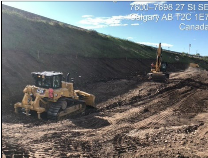
OGDEN - Preparatory work to construct the 78 Avenue diversion embankment.
