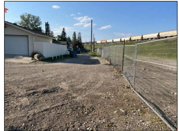
OGDEN – Safety fence installed between the work zone and residences.
