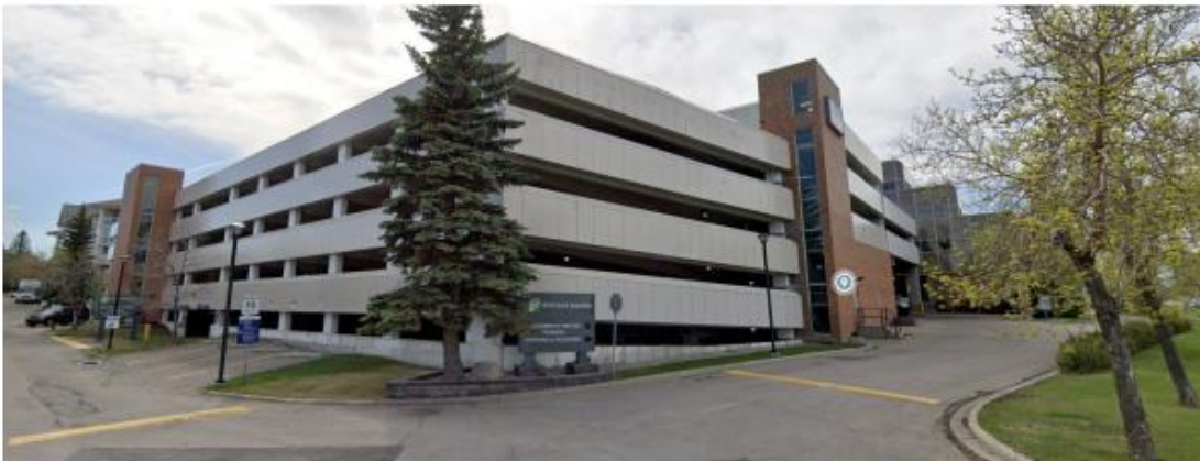
View south from private access road, showing parkade structure and north access
