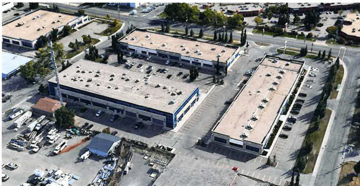
Arial View (North)
