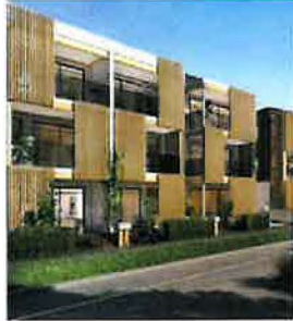
PRIVACY SCREENS FACING NEIGHBORS
